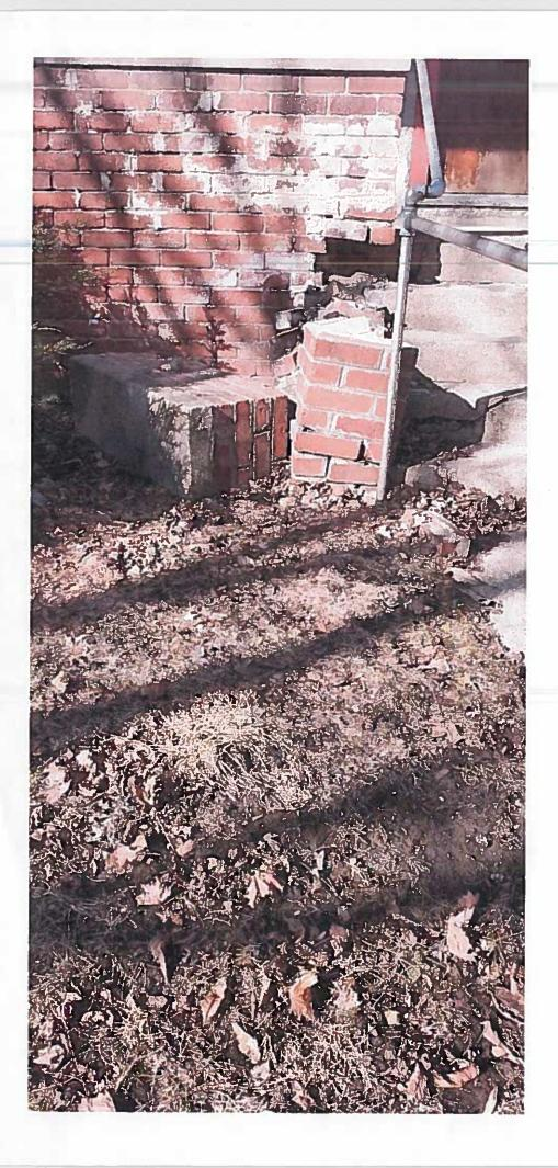
Repair and tuck point brick. Will be using the same material.
