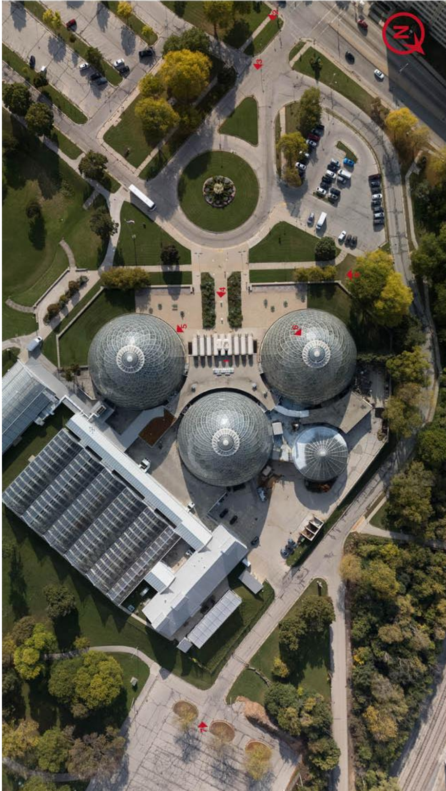
Figure 4: Site and Exterior Photo Key
