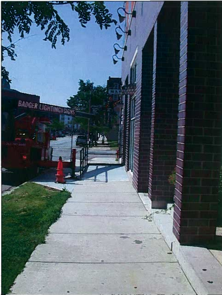
CCF 090262 1401-07 N Martin L King Jr Dr 8-13-09 Looking S towards W Vliet St at new ramp with handrail
