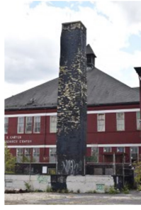
Photo7 North elevation of 1884 boiler house at
