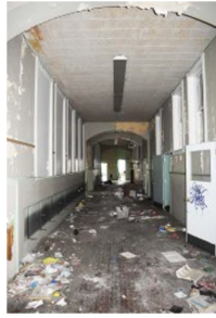
2nd floor 1898 block corridor -
