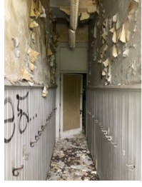
1st floor 1888 block typical cloak
