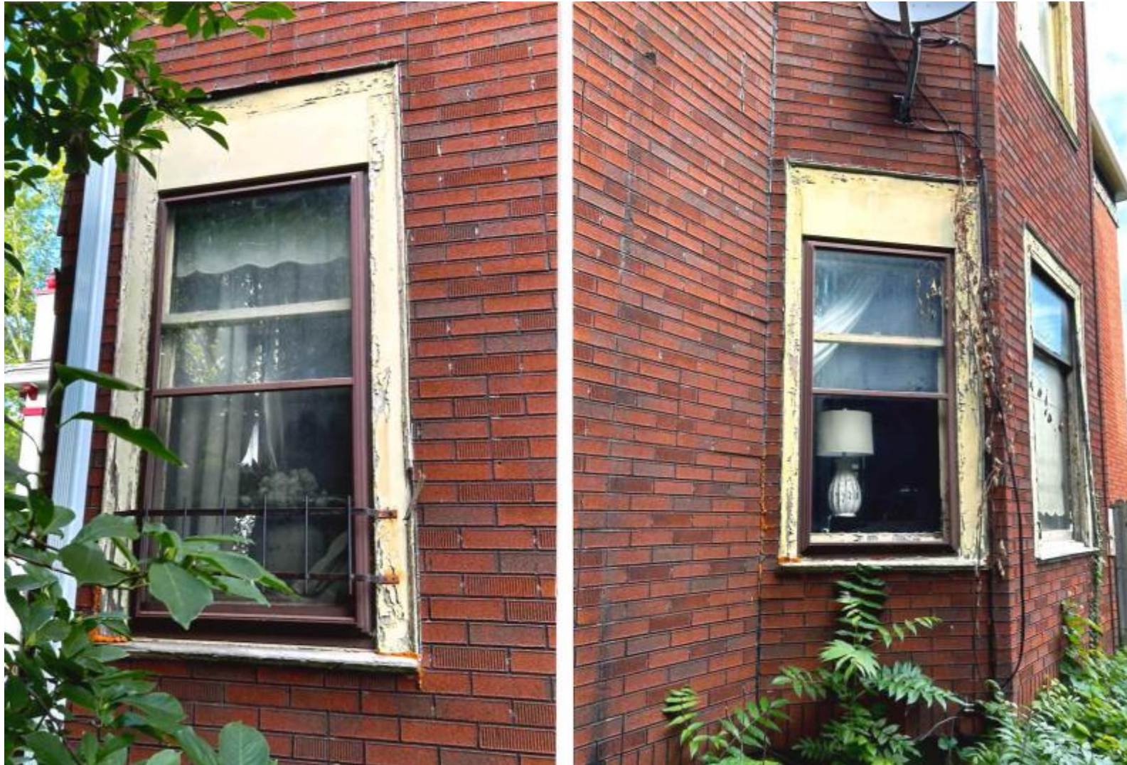
Prime windows to be repaired and restored and new wood storm windows installed
