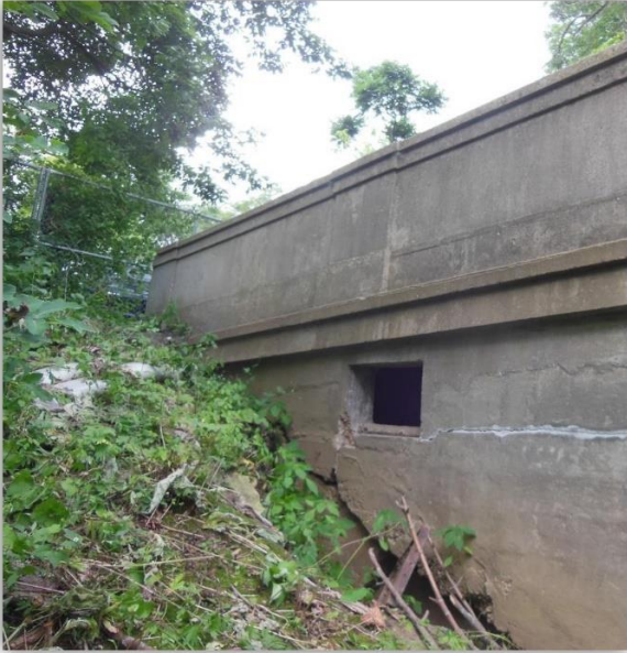
South wingwall with fractured wall exterior.
