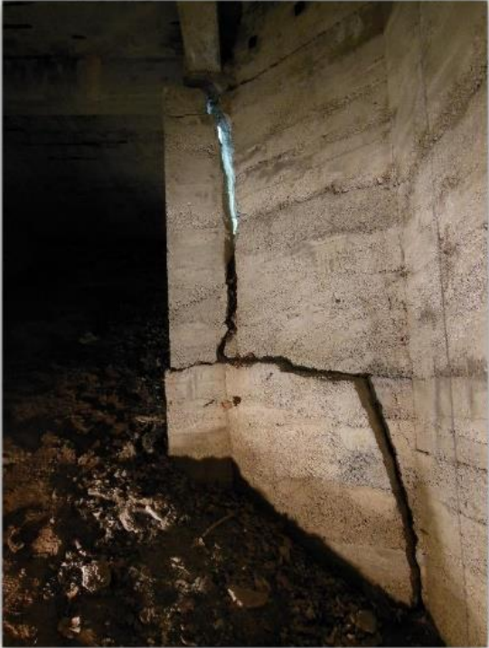
North wingwall (exterior and interior) with fractured wall.
