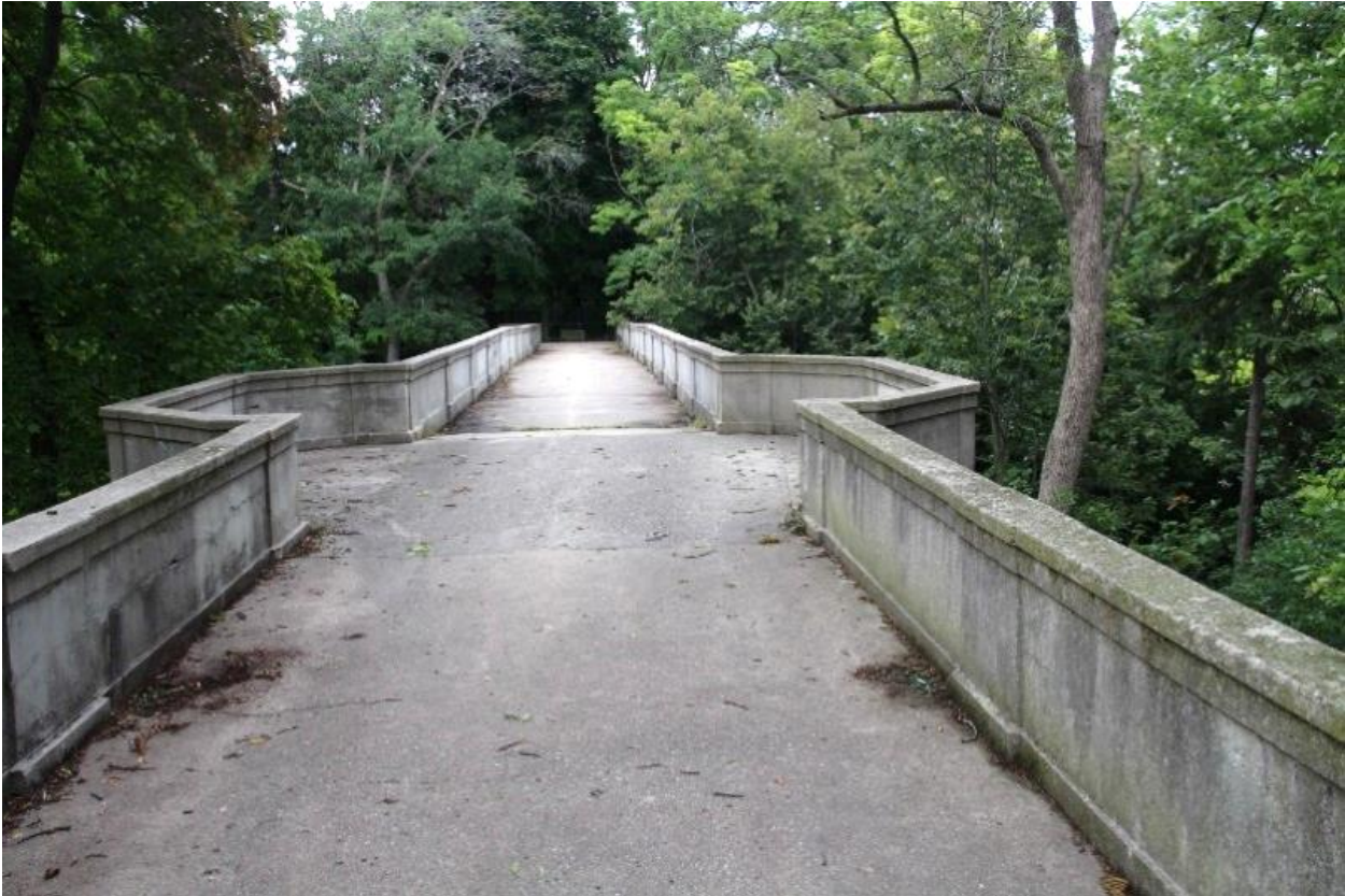
Overview of deck showing the alcove refuge over the abutment.
