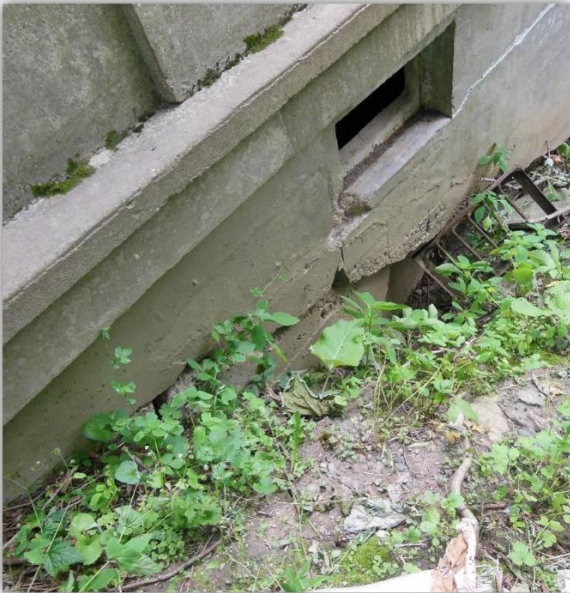
South wingwall with fractured wall exterior.
