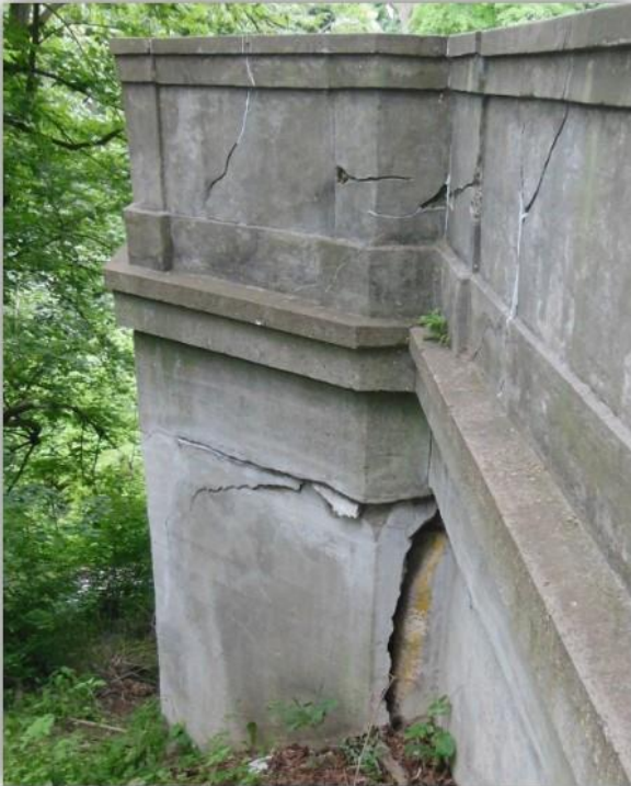
North wingwall (exterior and interior) with fractured wall.
