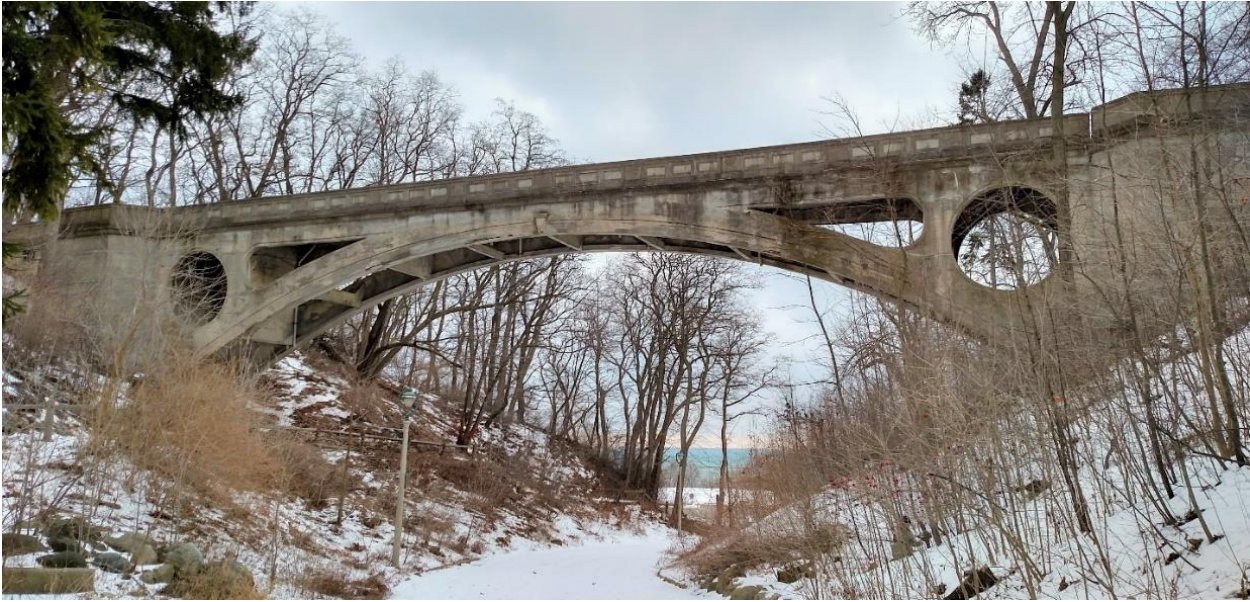
Overview image of the Lake Park Arch Bridge, view facing east.
