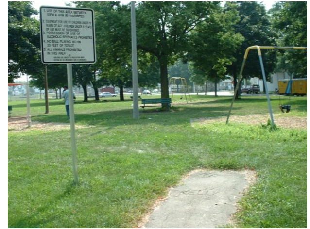
Example of inaccessible site entry
