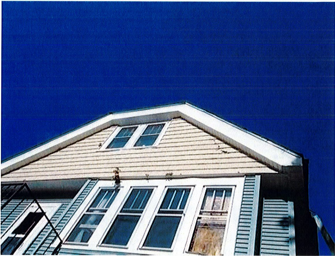
27-Front Elevation Close up of metal shake siding
