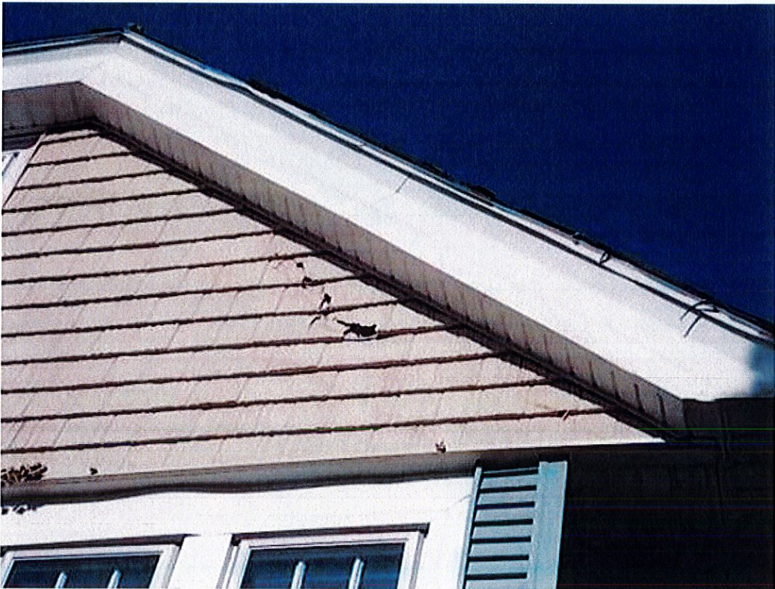
26-Front Elevation Close up of metal shake siding
