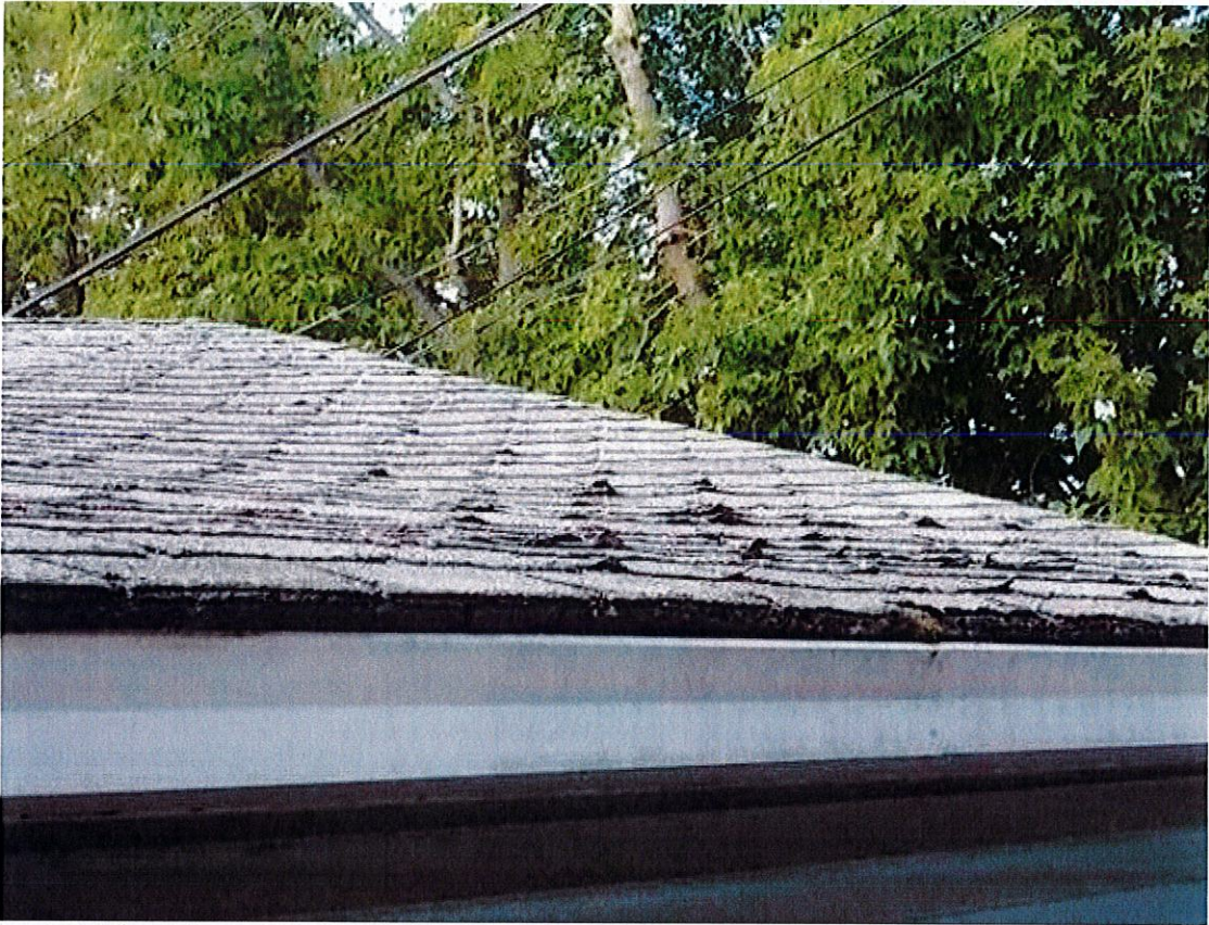
39-Detached Gargae NO damage to the organic shingles.
