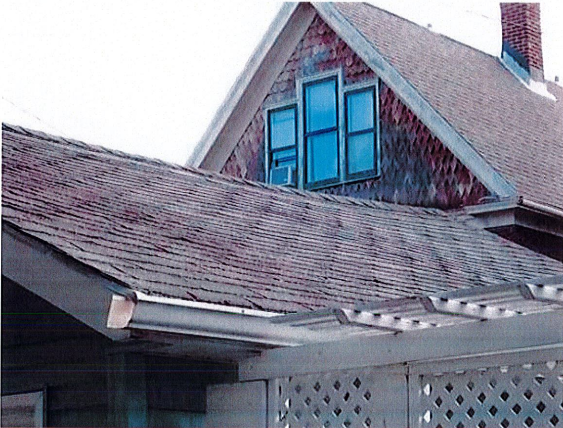
40-Detached Gargae NO damage to the organic shingles.
