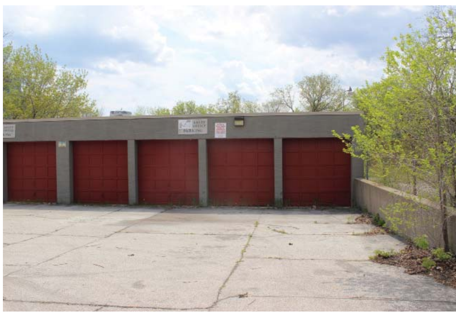
Block A existing structure
