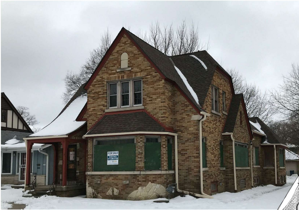
PHOTO OF CURRENT CONDITIONS
