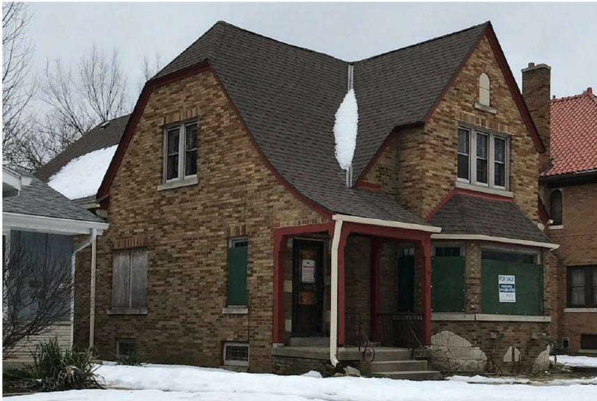
PHOTO OF CURRENT CONDITIONS
