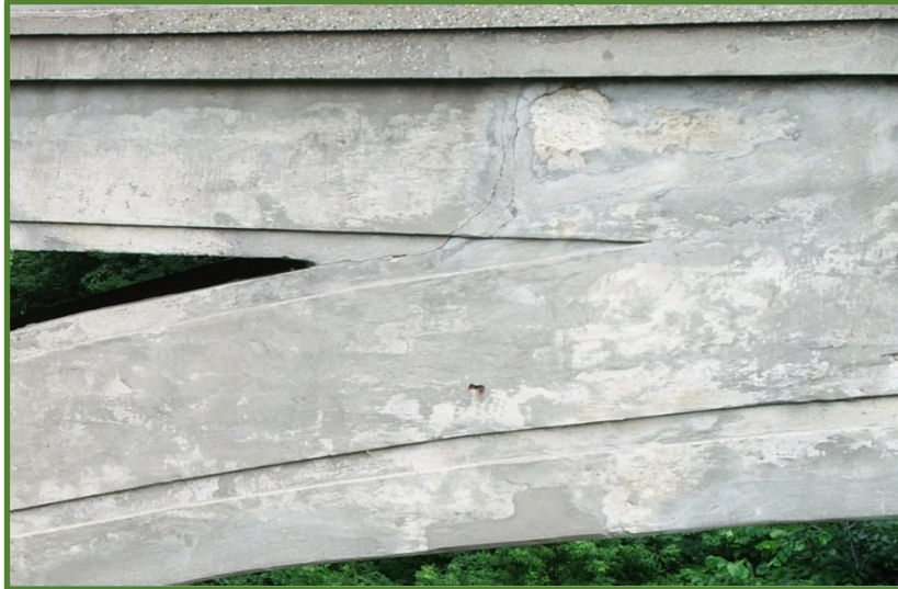
Figure 5: East Arch Rib and Spandrel Face w/ Parge Coat
