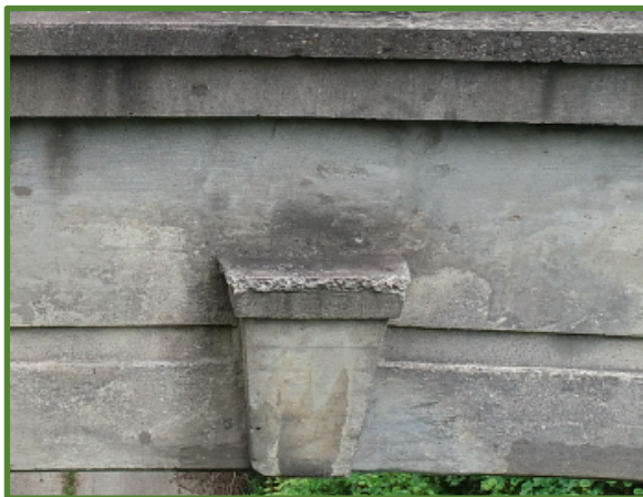
Figure 2: Arch Rib Finial
