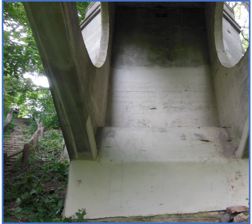
Figure 1: North Thrust Block Shotcrete Face
