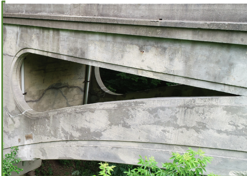
Figure 6: West Arch Rib & Spandrel Wall Face w/ Parge Coating
