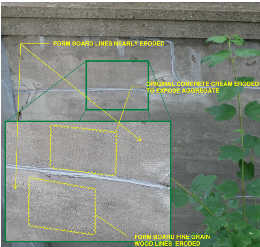
Figure 4: Existing Original Concrete Surface
