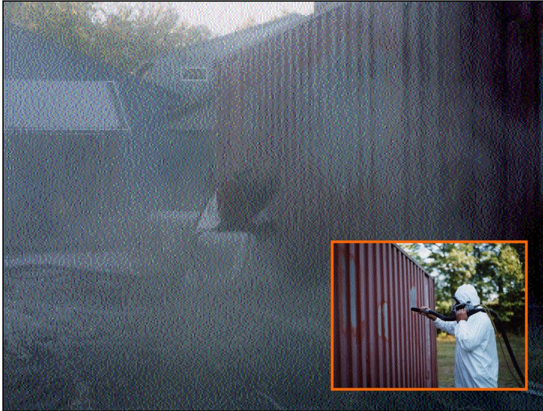
Blasting with Sponge Media™ abrasives can reduce dust levels as much as 99.9% when compared to traditional abrasive blasting.
