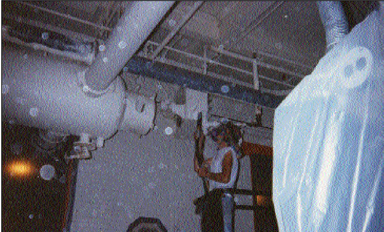
Sponge Media abrasives reduce rebound energy causing less damage to surrounding surfaces and sensitive machinery.
