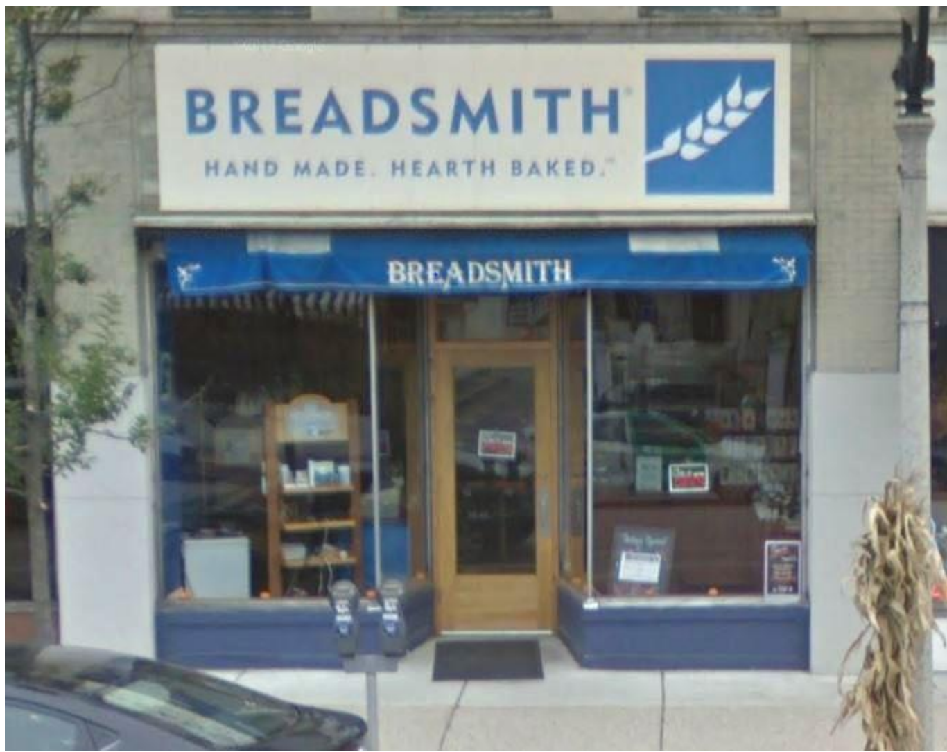
Image of existing storefront
