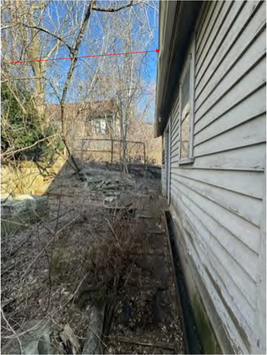
North Face of Rear House
