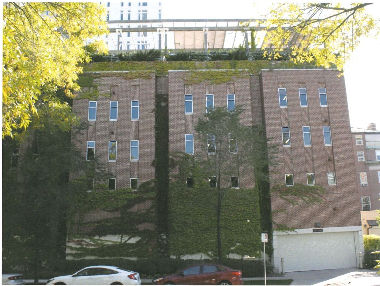
1 CONTEXT, EAST P1.3 UNIVERSITY CLUB, PARKING GARAGE
