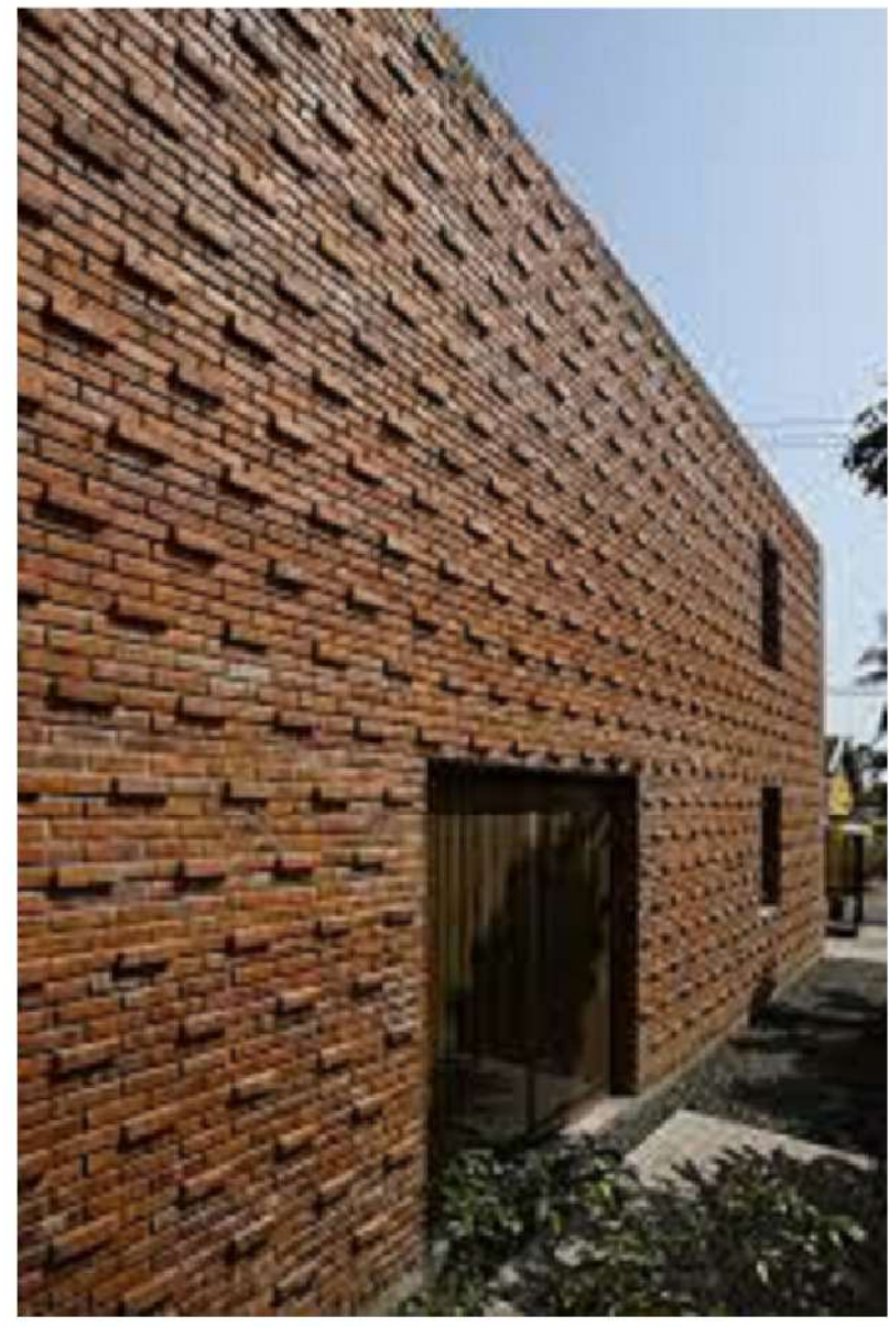
EXAMPLE OF BRICK ACCENT (SEE EXTERIOR ELEVATIONS & CORRESPONDING KEY NOTE 8)
