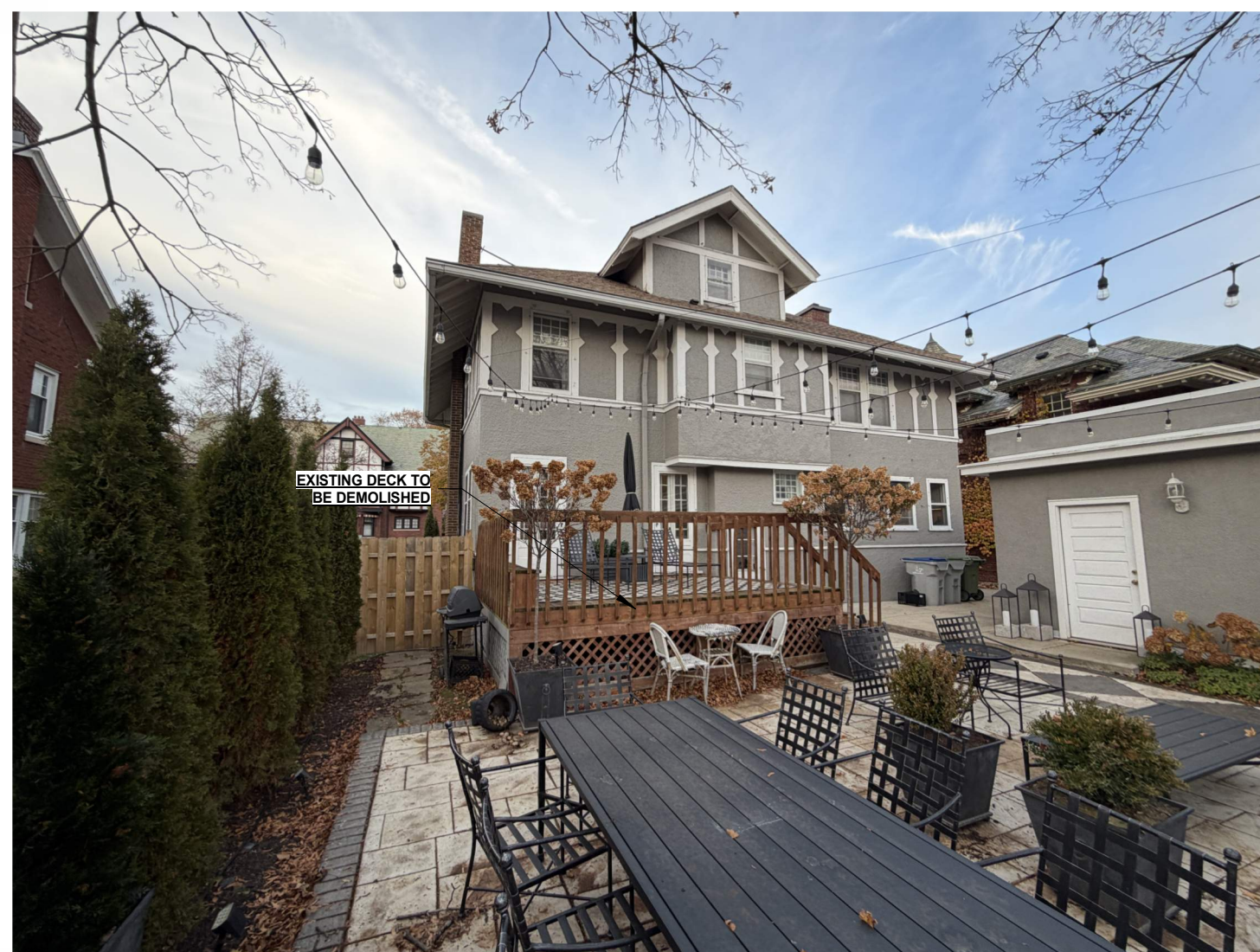
EXISTING CONDITION PHOTOGRAPH
