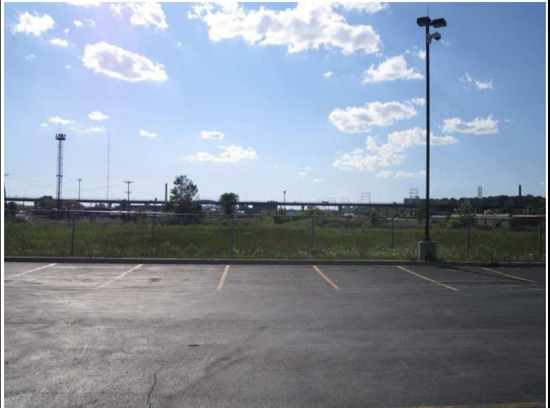
West View from Biogas Generation Site
