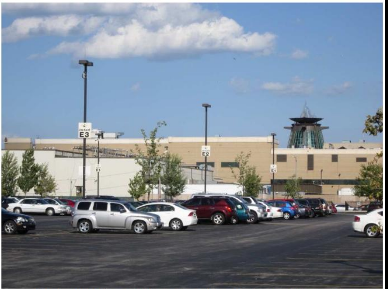
East – Northeast View from Biogas Generation Site
