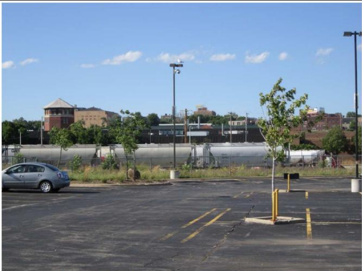
North View from Biogas Generation Site
