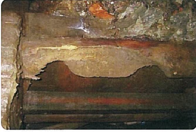
Wood Pile Underpinning Repairs - Boston, MA
