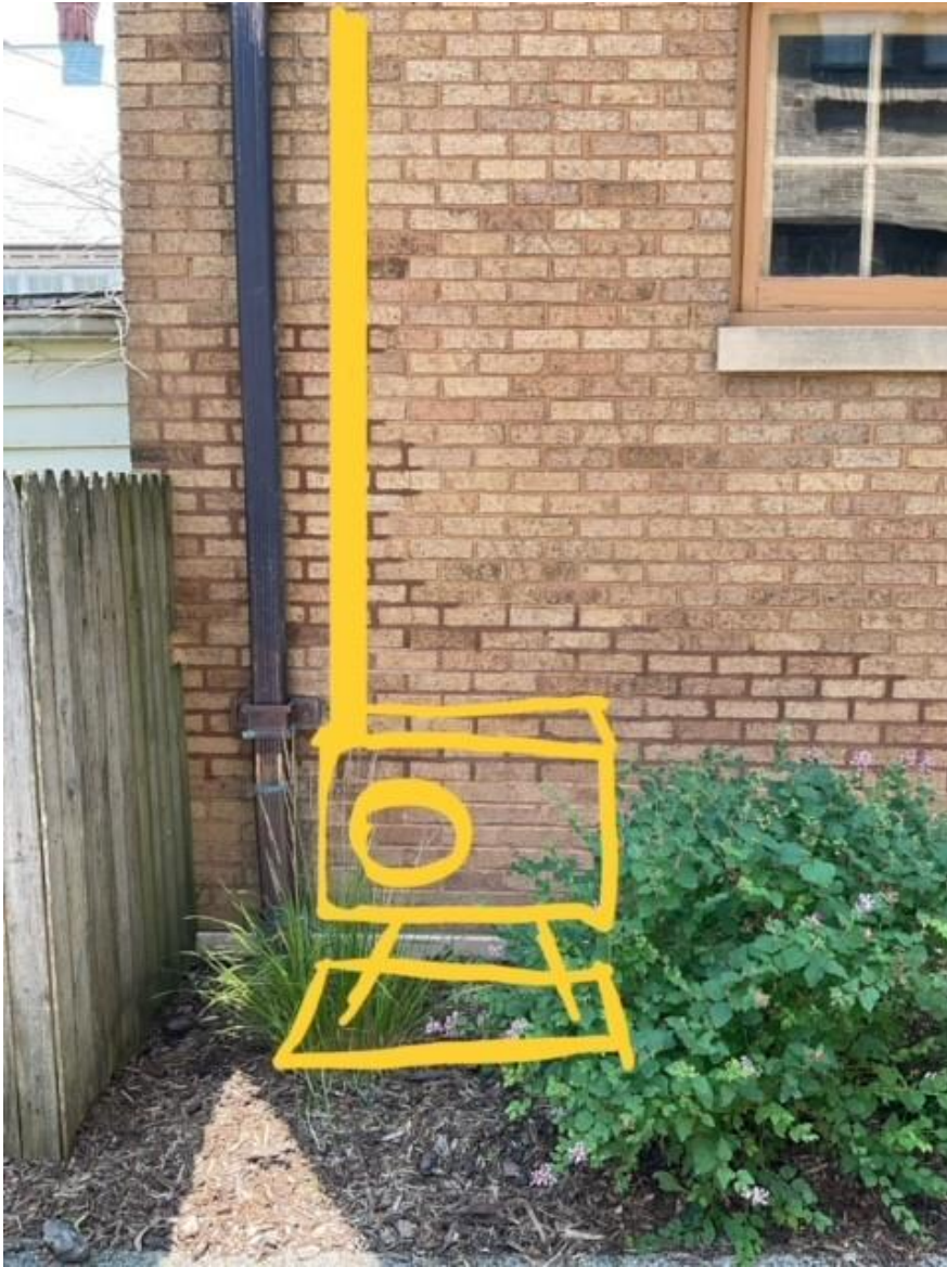
Location of HVAC equipment at rear facade
