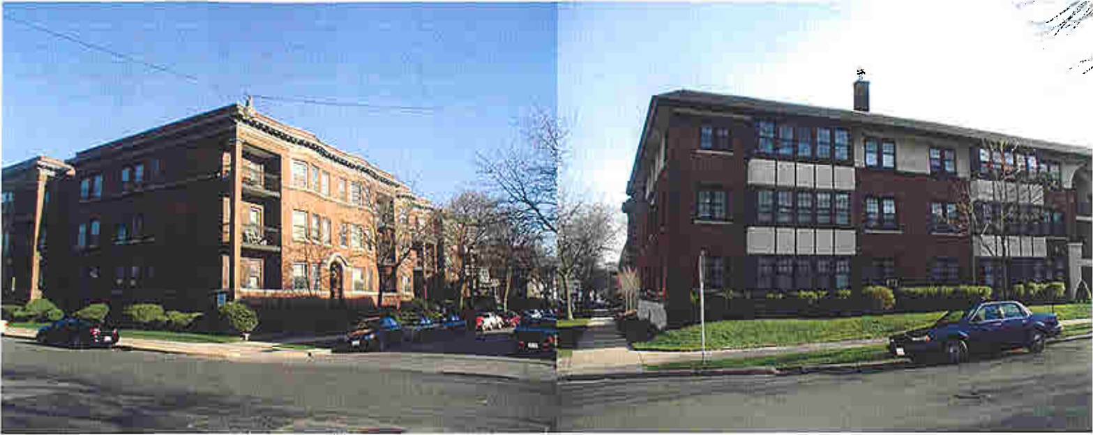
1. VIEW SOUTH ON STOWELL AVE.
