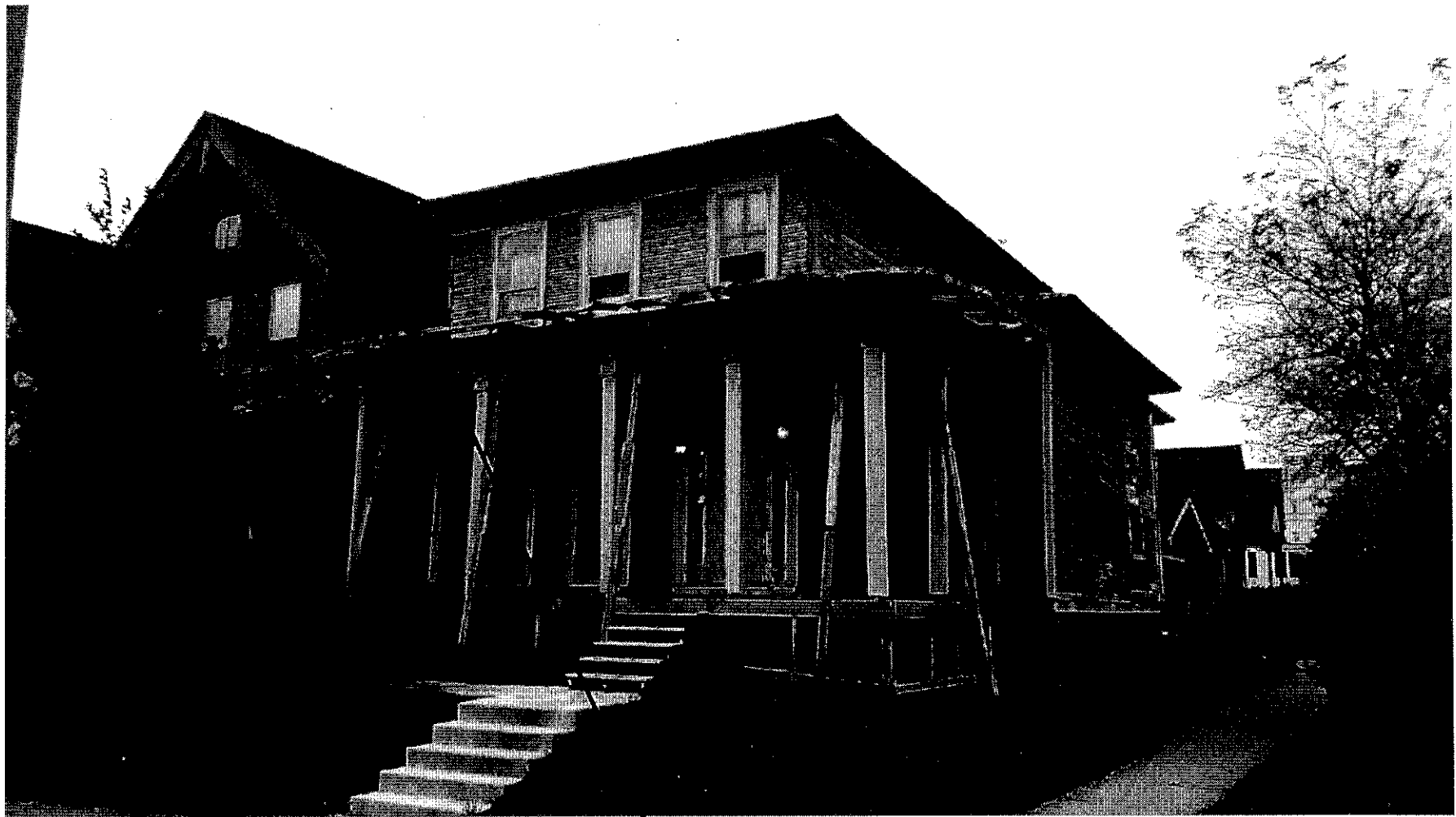
Current photo (10/3/14) of house showing partially rebuilt porch with extensive deterioration to fascia, soffit, ceiling and roof decking. Previous attempt to rebuild porch utilized common pine boards with knots. This must be replaced with clear, knot free material. The finish material on the building now exhibits extensive mold coverage.
