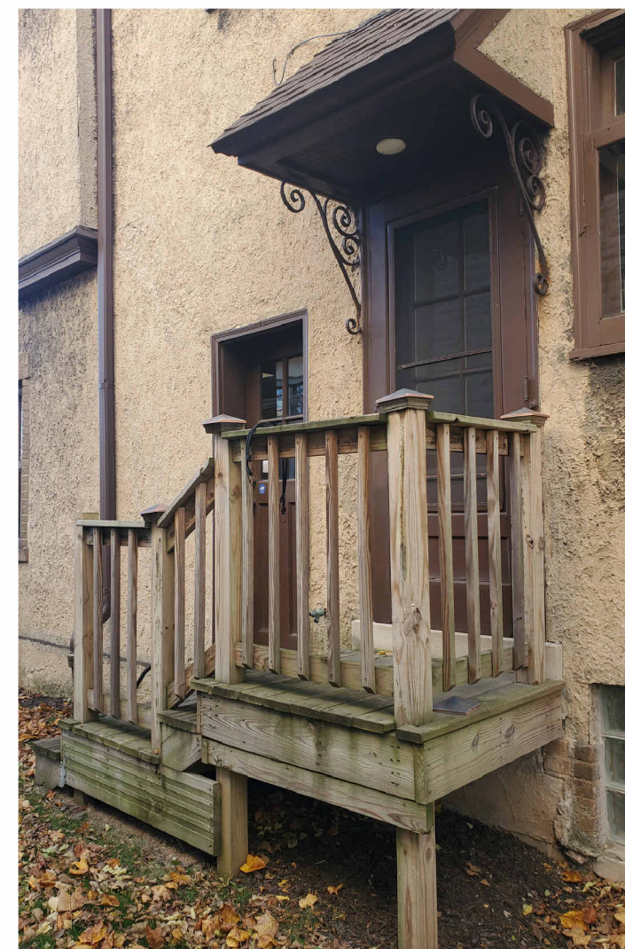
8 Existing North Stair 3/16" = 1'-0"
