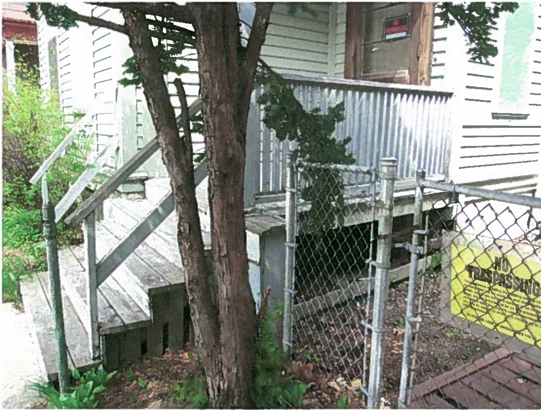
3. First Floor (South-East Elevation) with horizontal stair railing and missing porch skirt
