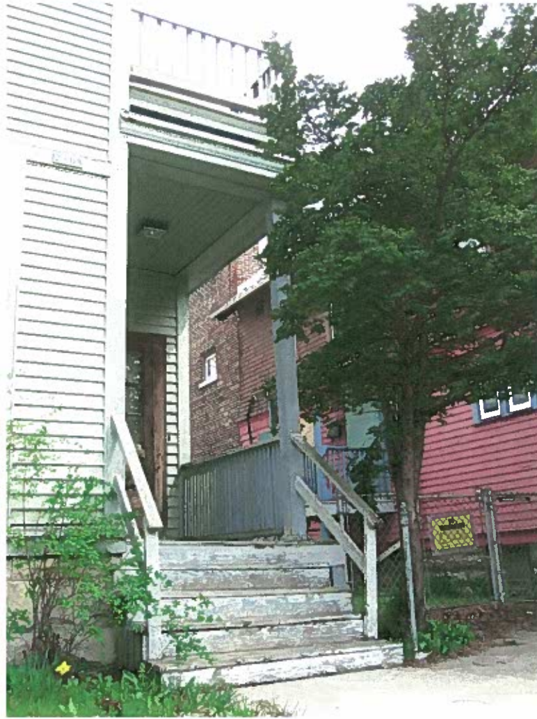
1. Front Porch (South Elevation)
