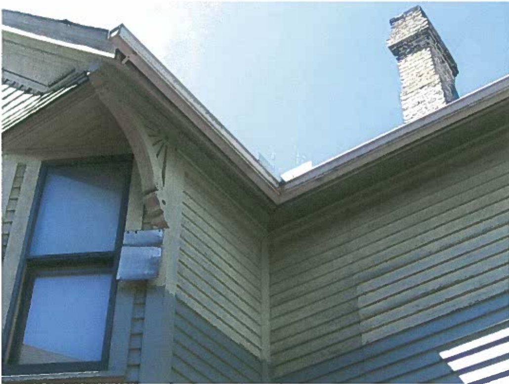
7. Second floor (North-East Elevation) above side porch
