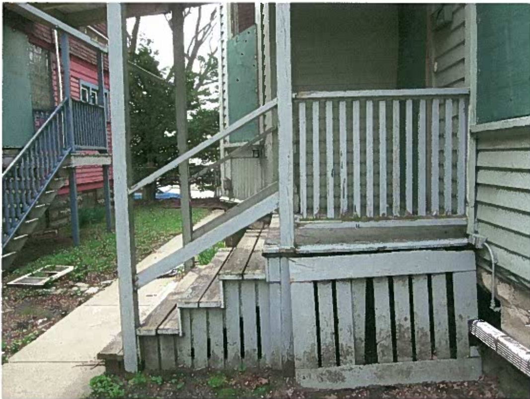
10. Side porch (North Elevation)
