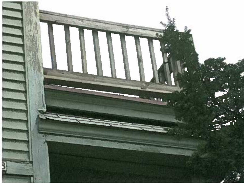
2. Upper deck railing above front porch
