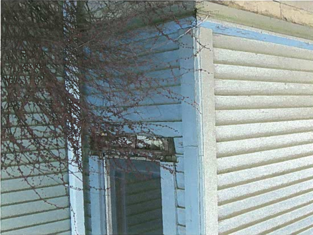
11. Front side window (South-West Elevation) with missing Stool and Apron
