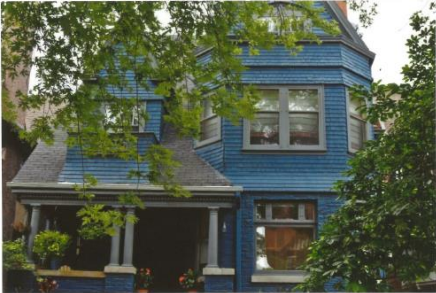
Current condition of the property Front (southwest) Elevation
