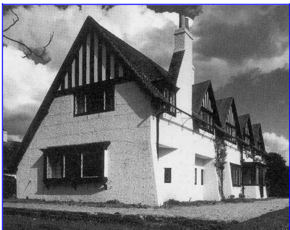
Walnut Tree Farm (1890) in Castlemorton, Hereford and Worcester, England. Designed by C. F. A. Voysey, this cottage employs a sweeping roof (also called a cat slide roof) that is one hallmark of the Arts and Crafts style and also a pivotal design feature of the Manegold house in Milwaukee.
