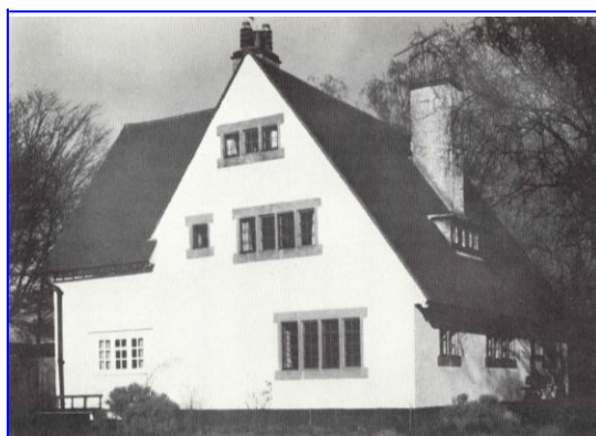
Stanley Parker Cottage (1908) designed by Parker and Unwin for the renowned Letchworth Garden City development in England. Roughly contemporary with the Manegold house in Milwaukee, it incorporates many of the details of Voysey's earlier Arts and Crafts design work. Parker and Unwin's work was highly influential with architects in America.
