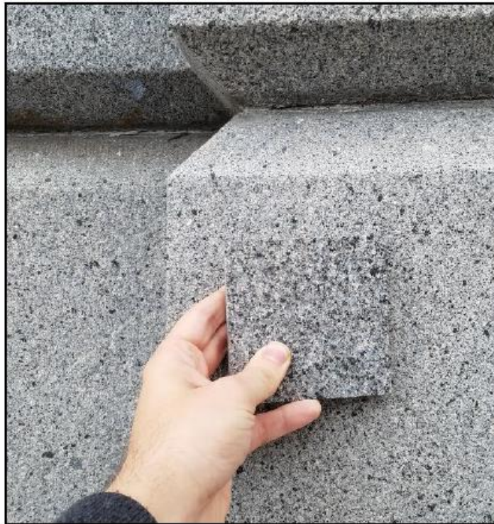
MASONRY VENEER 2 HALQUIST STONE – CHARCOAL THERMAL
