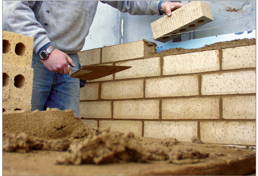
Consistent custom colored mortar, every time
