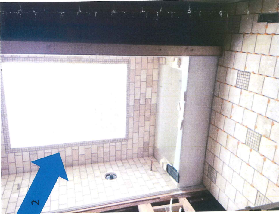
1.) Existing glass-block window saved and flanked with travertine tile, as part of bathroom renovation; including new plumbing, electrical, lighting, vent, HVAC, walls, travertine tile, vanity, sink, bathtub, toilet, doors, and brushed nickel finishes.
