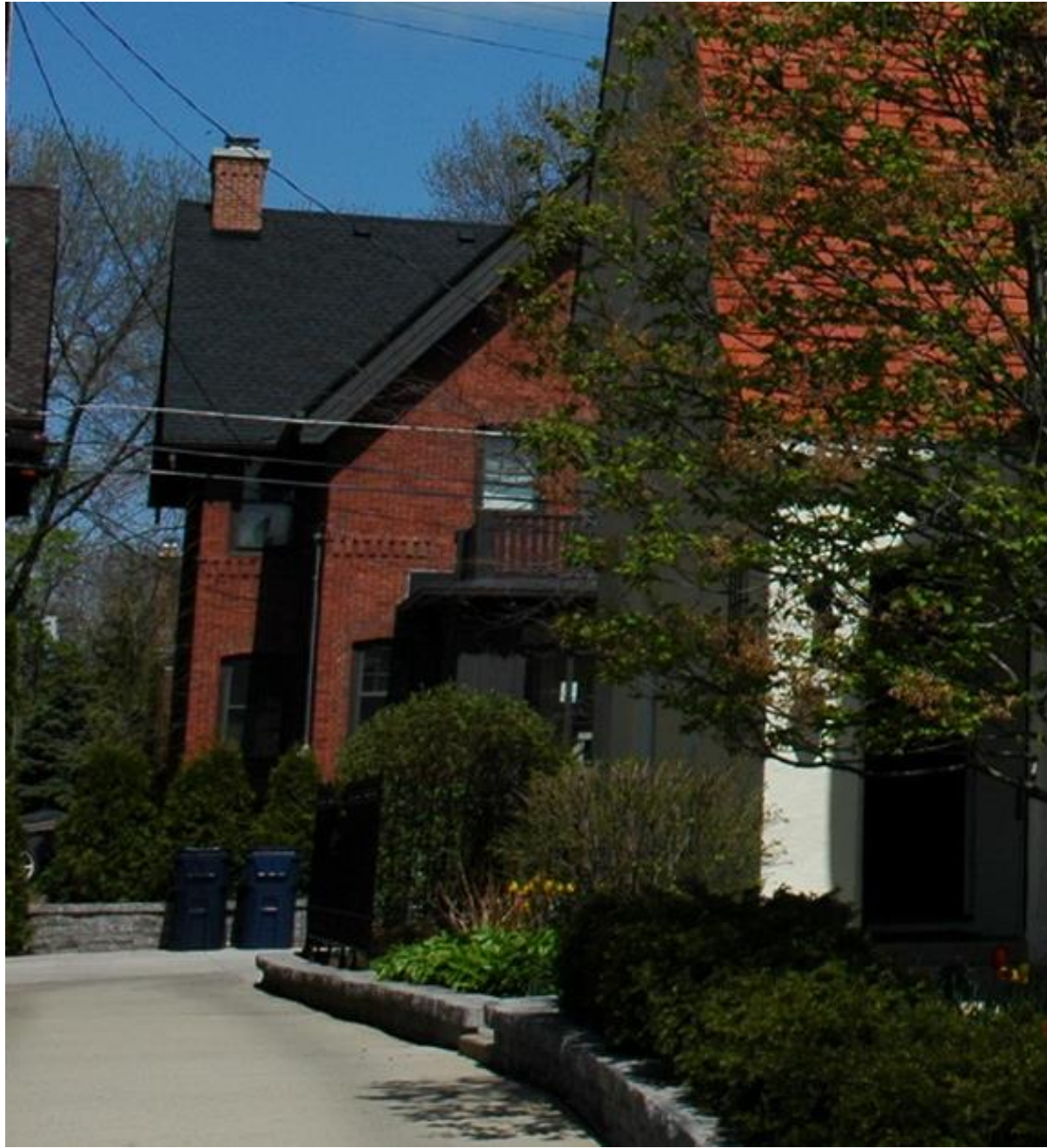
Previous railing c. 2010.
