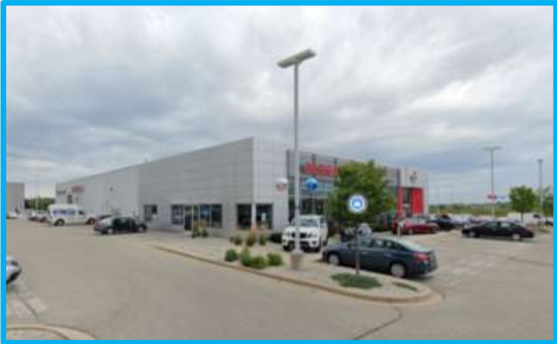
View of lobby entry, looking northwest
