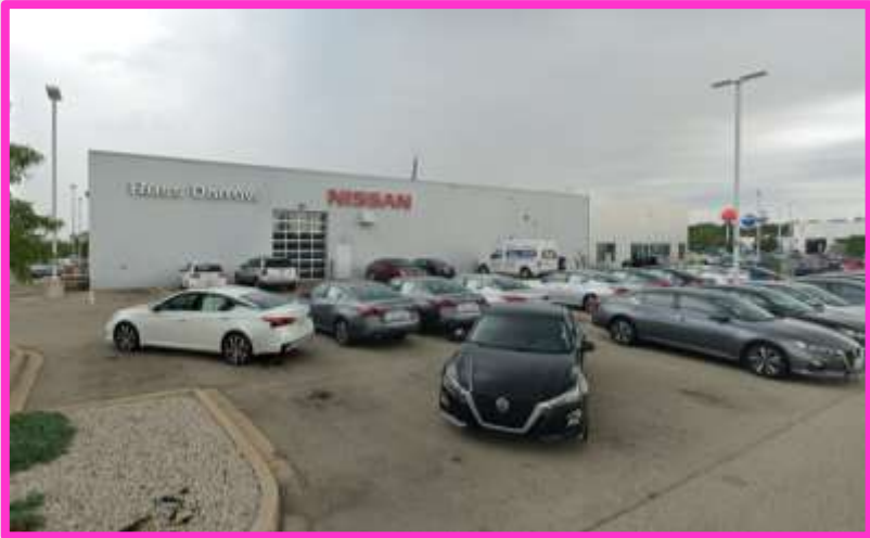
View looking north, location of proposed building addition
