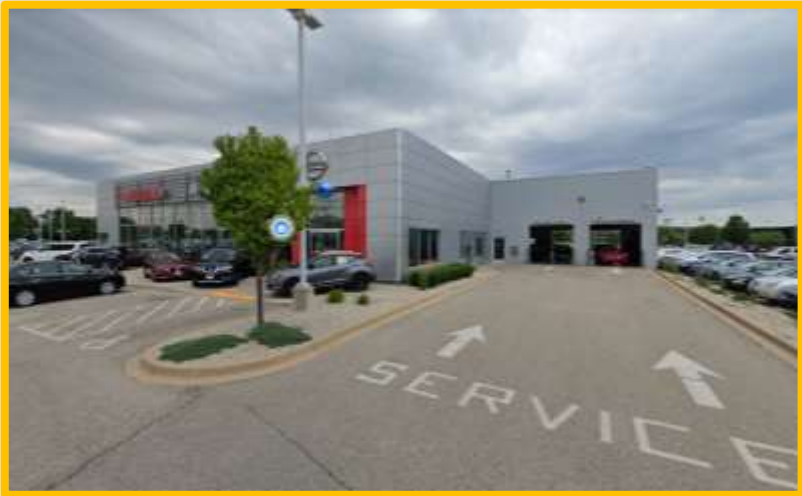
View of service and lobby entries, looking west
