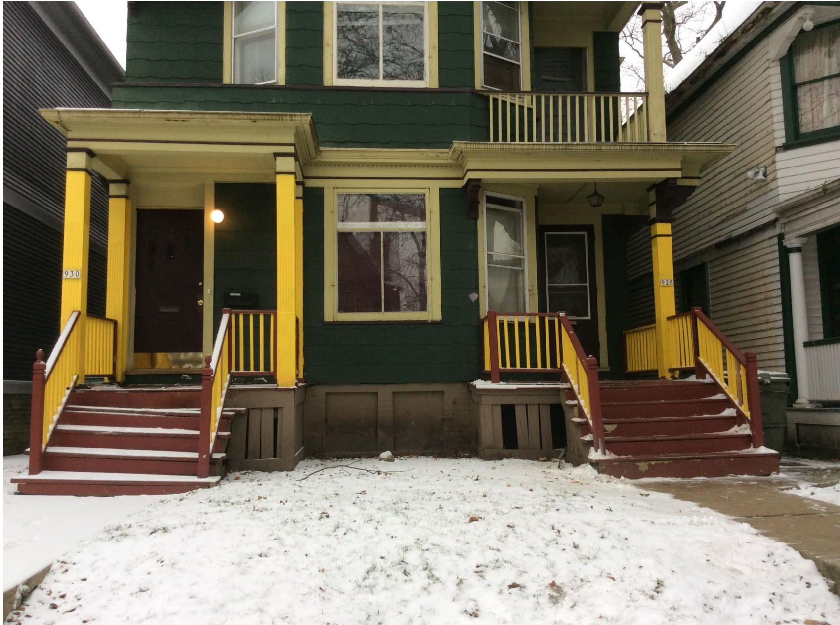
2018 photo. Columns are to remain as existing.
