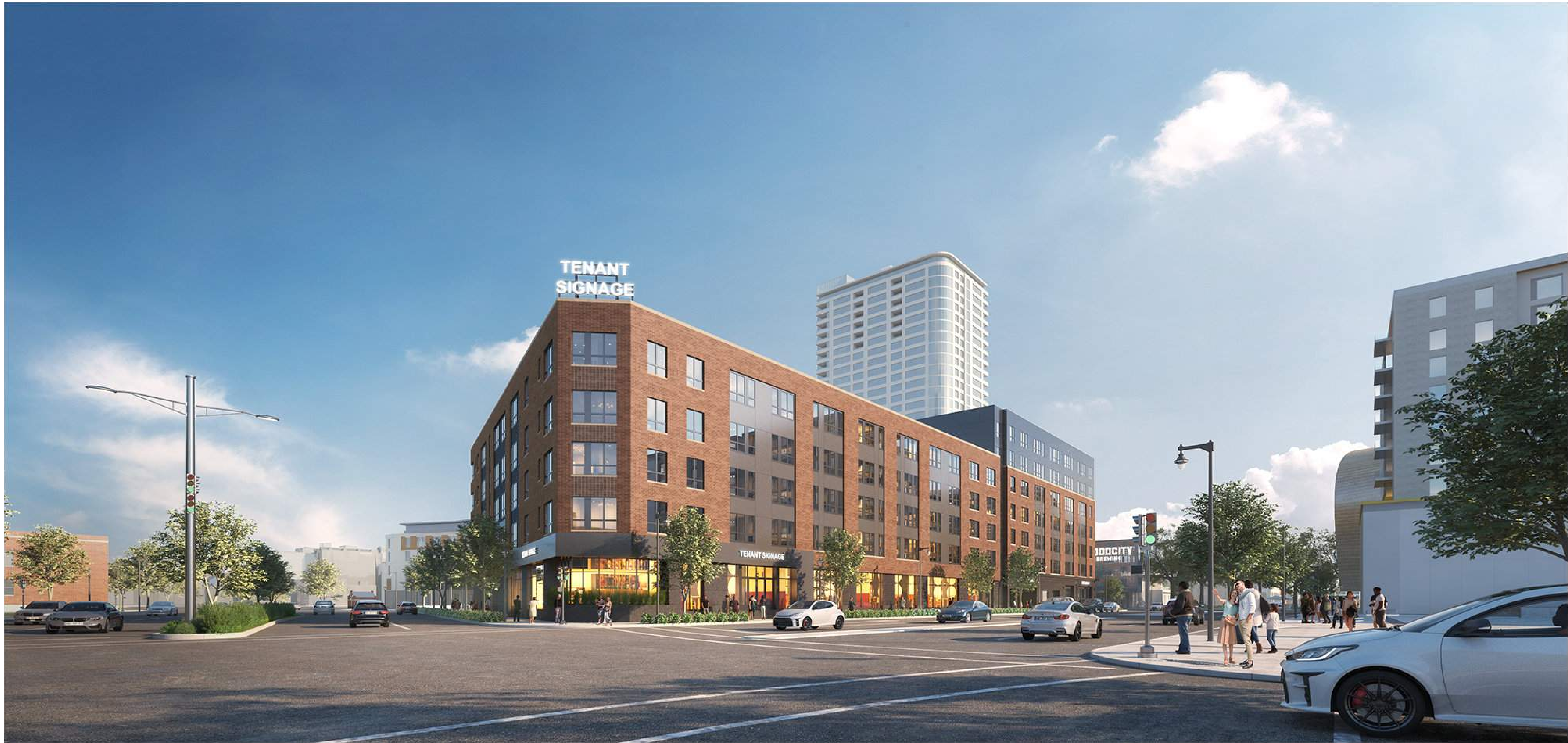
VIEW OF NORTHWEST CORNER
