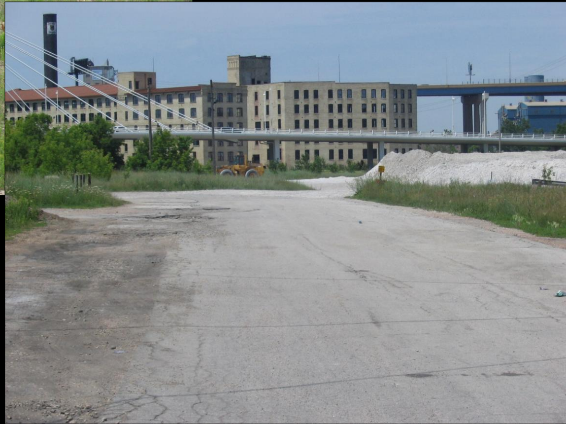
Bottom: Looking West from W Oregon St in the Reed Street Yards
