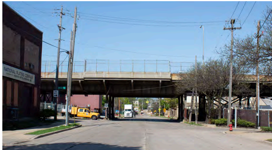
Image above shows the view from W. Bruce Street, looking west, under the N. 16th Street viaduct. Stakeholders agree this location is in need of lighting, safety, and aesthetic enhancements.
