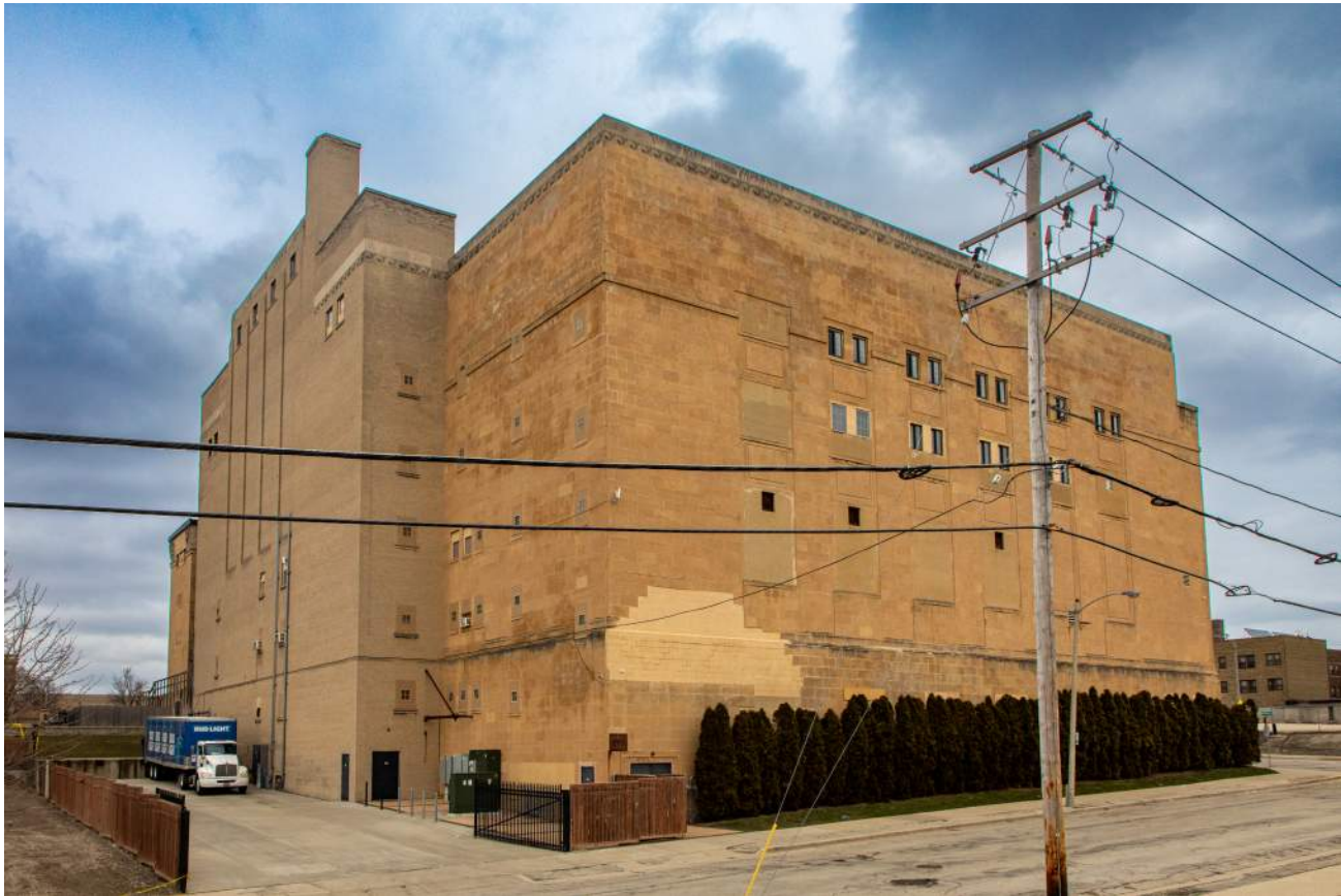
Photo 5 - South West Elevation
