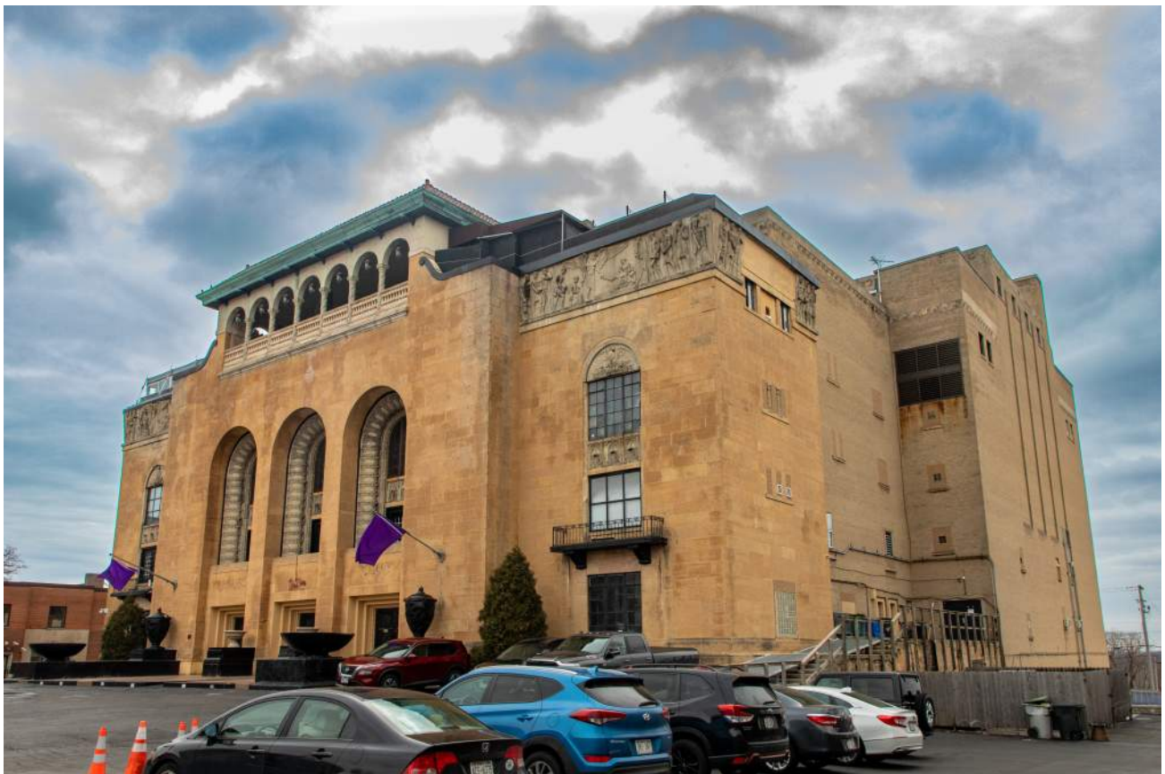
Photo 2 - North West Elevation
