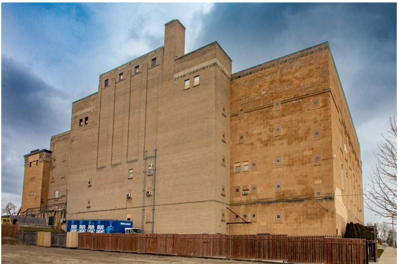
Photo 4 - South West Elevation
