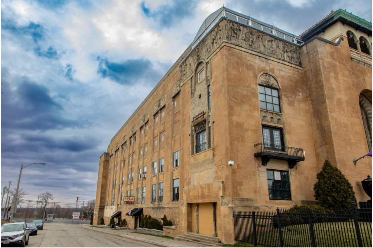
Photo 9 - North East Elevation
