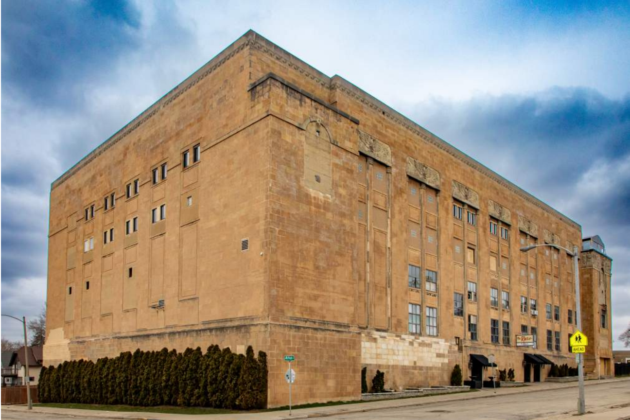
Photo 7 - South East Elevation
