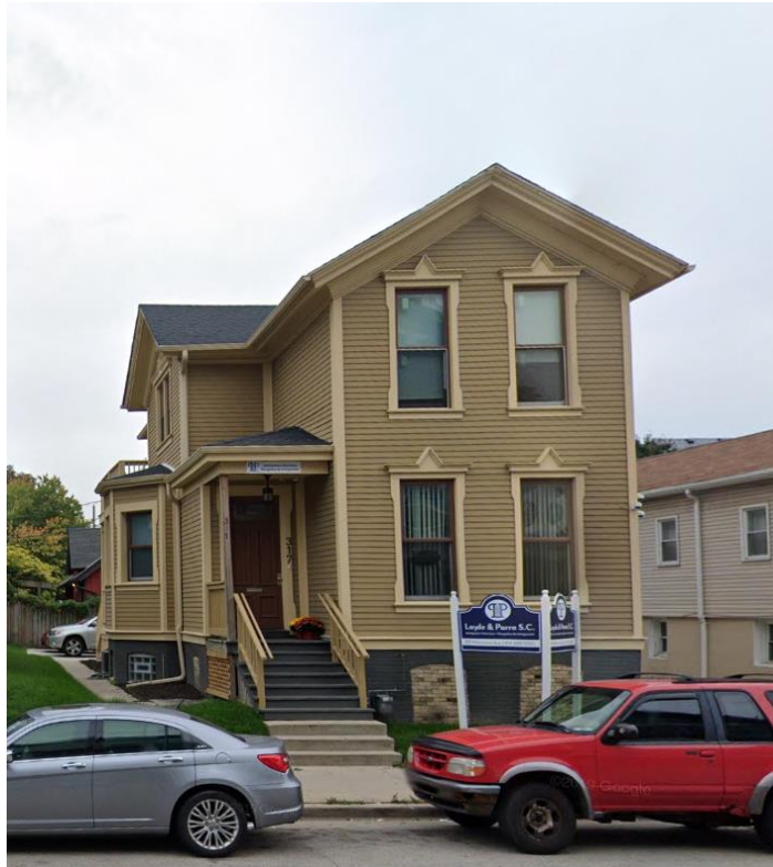
317 West National, front facade
