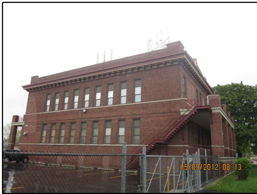
EXISTING BUILDING ELEVATION & ANTENNAS
