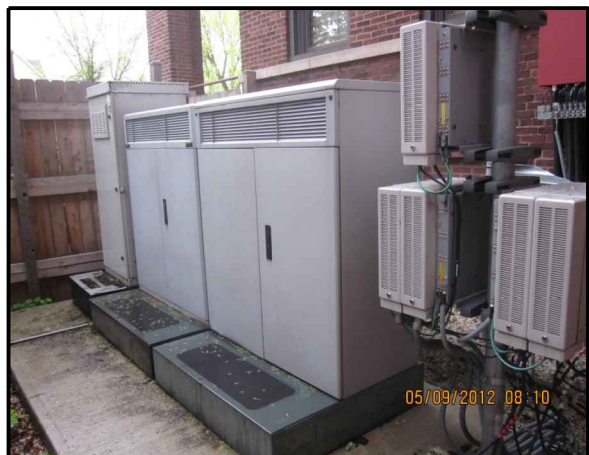
1 C-2 EXISTING SITE OVERVIEW [LOOKING NW]
