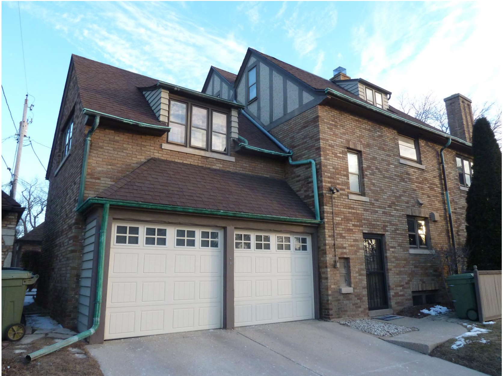
Replacement doors in February 2017
