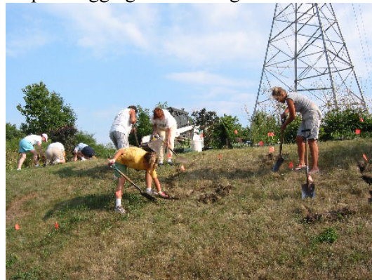
Step 2: Digging & trenching
