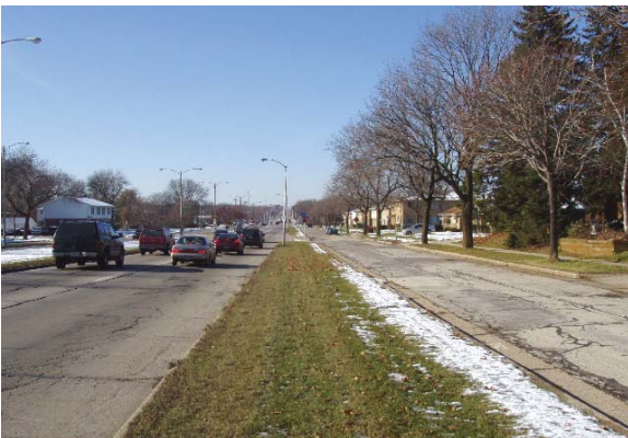
Oklahoma Ave. and frontage road
