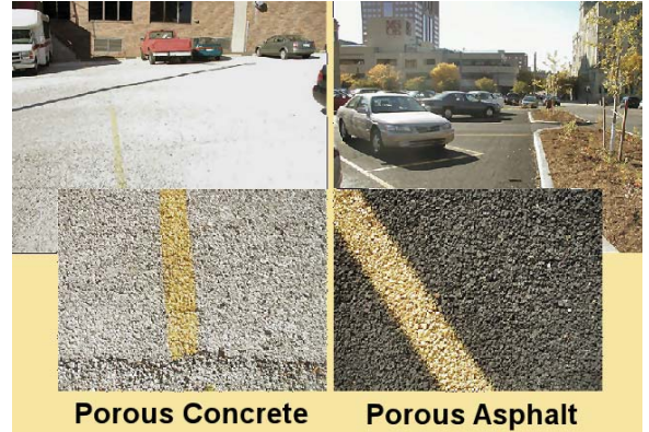
Porous pavement at Milwaukee School of Engineering Source: Milwaukee Department of Public Works website
