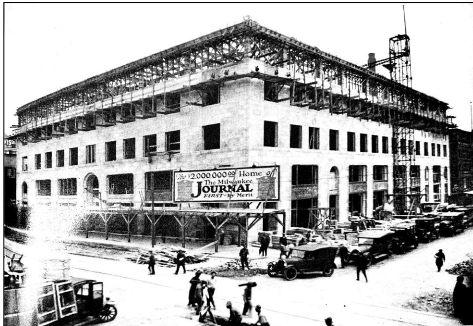
Figure 4 of 28: Historic photo of the 1924 Milwaukee Journal Building under construction, c, 1924. Source: The Milwaukee Journal, An Informal Chronicle of Its First 100 Years.
