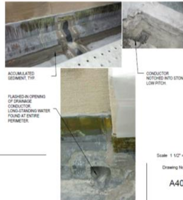
2 CORNICE FLASHING, DRAIN - SECTION DETAIL 1 1/2" = 1'-0"
