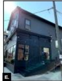
Continue Historic Details at Deck: Replace existing trim, corbels and pilasters at new exterior deck. Paint new trim to match existing finish scheme.
