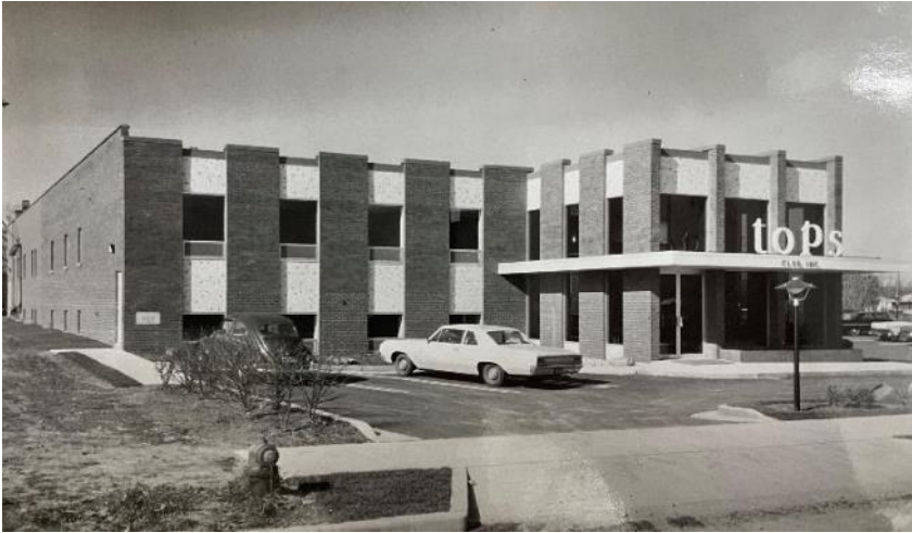
PHOTOGRAPH, SUMMER 1965. TOPS HEADQUARTERS UPON COMPLETION, EXTERIOR.
