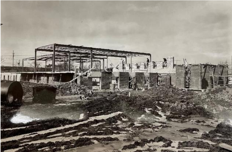
PHOTOGRAPH, SPRING 1965. TOPS HEADQUARTERS UNDER CONSTRUCTION.
