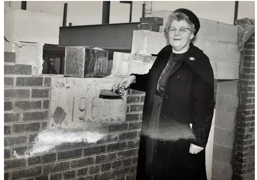
PHOTOGRAPH, SPRING 1965. ESTHER MANZ AND CORNERSTONE DURING CONSTRUCTION.
