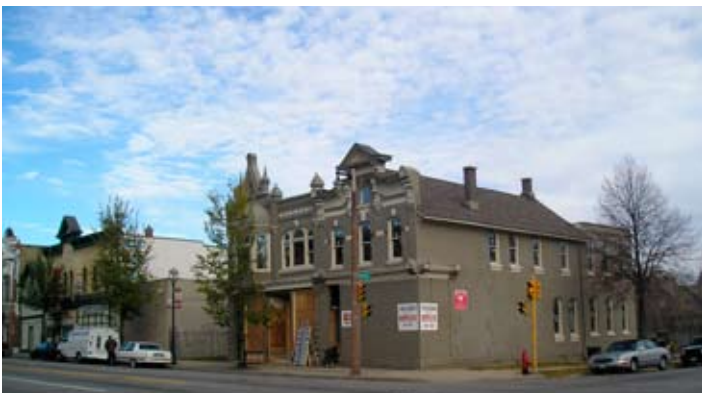
Figure 7.26: Center Street and Holton Street - Existing Conditions
