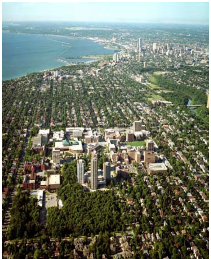
Figure 9.3: Aerial of UWM campus in foreground and neighborhoods to the south.
