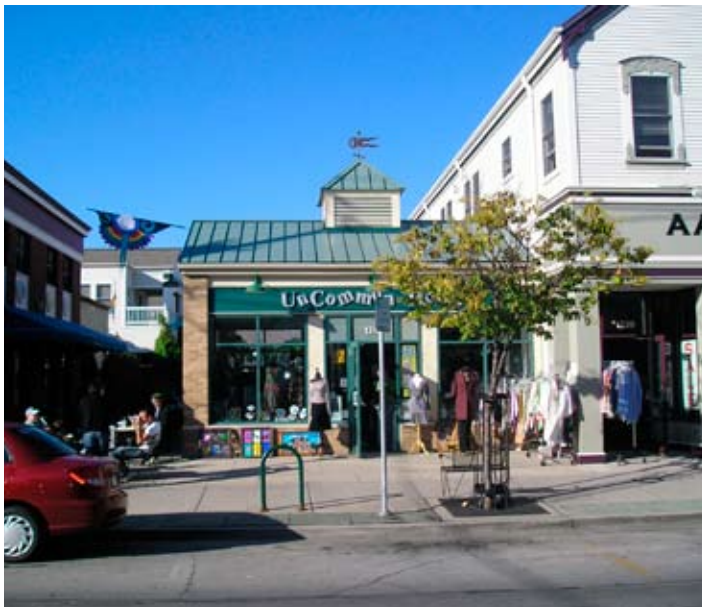
Figure 2.28: Brady Street Retail - Passeggio Complex
