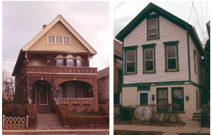
Figure 10.15: Historic housing stock in the East Village Historic District.
