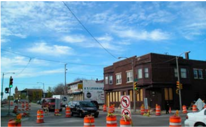
Figure 7.25: Center Street and Holton Street - Existing Conditions
