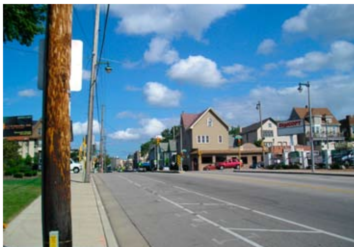
Figure 10.10: Brady Street looking east at areas of potential redevelopment.
