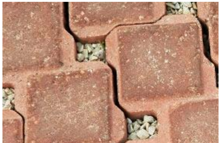
Figure 3.20: Josey Heights Porous Pavers
