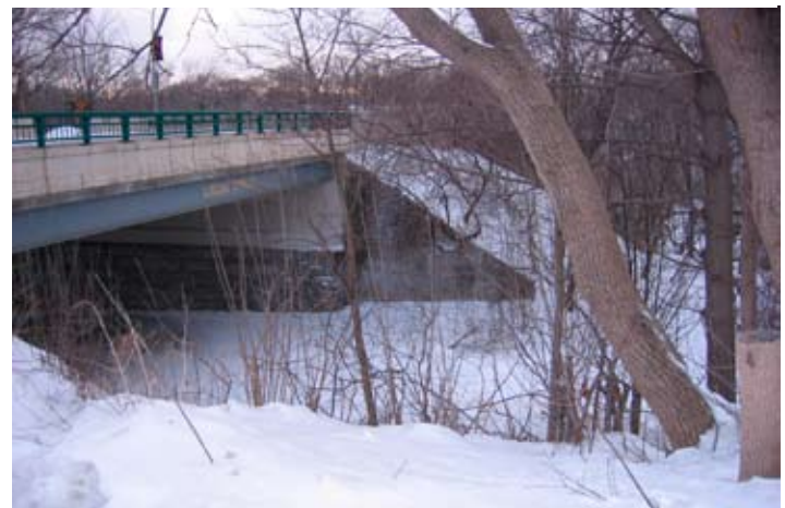
Figure 8.22: Bridge Over Oak Leaf Trail at Locust Street
