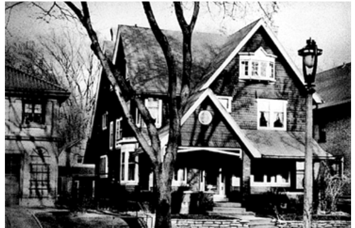
Figure 1.20: 1904 Arts and Crafts house, Upper East Side Source: Historic Preservation Office, City of Milwaukee
