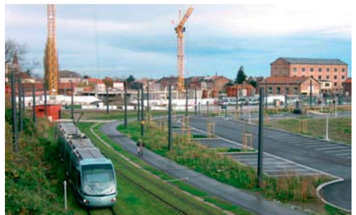
Tramway in Valenciennes. The urban landscape associated with the tramway can be used to increase the value of the areas through which they run: paving materials can be changed, trees can be planted and grass can be laid along the tramway tracks.
