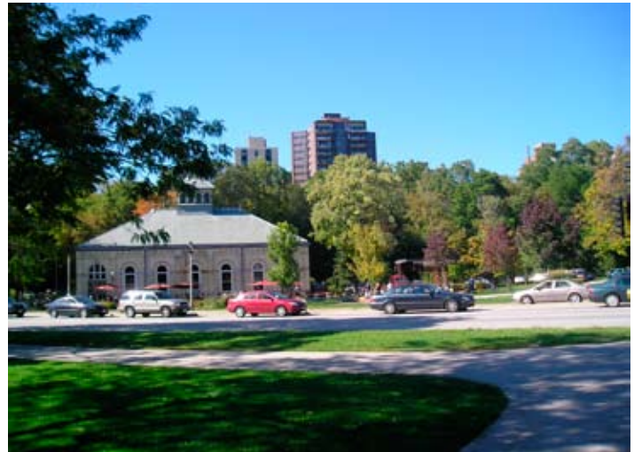
Figure 11.6: Alterra on the Lake Coffee Bar (former flushing station)
