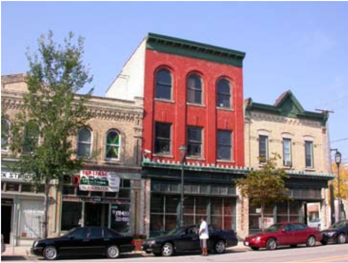
Figure 5.6: Historic King Drive
