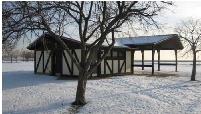
Figure 11.30: Existing Restrooms and Picnic Pavilion
