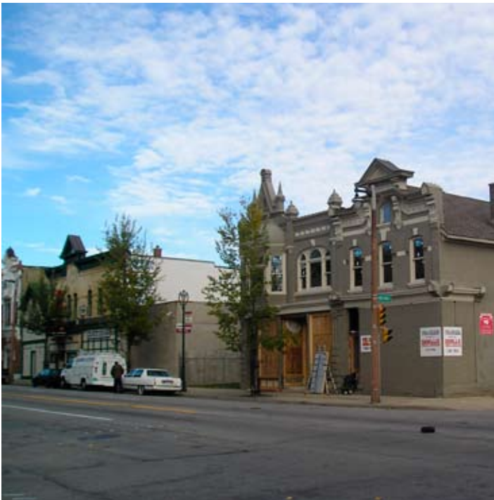
Figure 5.32: Vacant Property Available - Historic Potential (Historic facade in need of renovation.)
