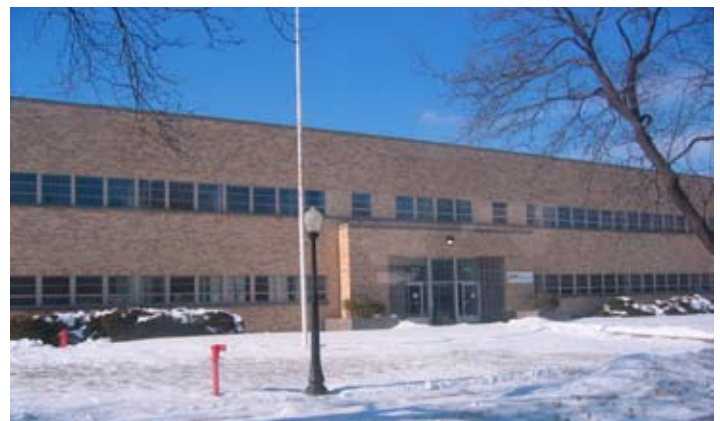
Figure 6.4: Existing Industrial Buildings
