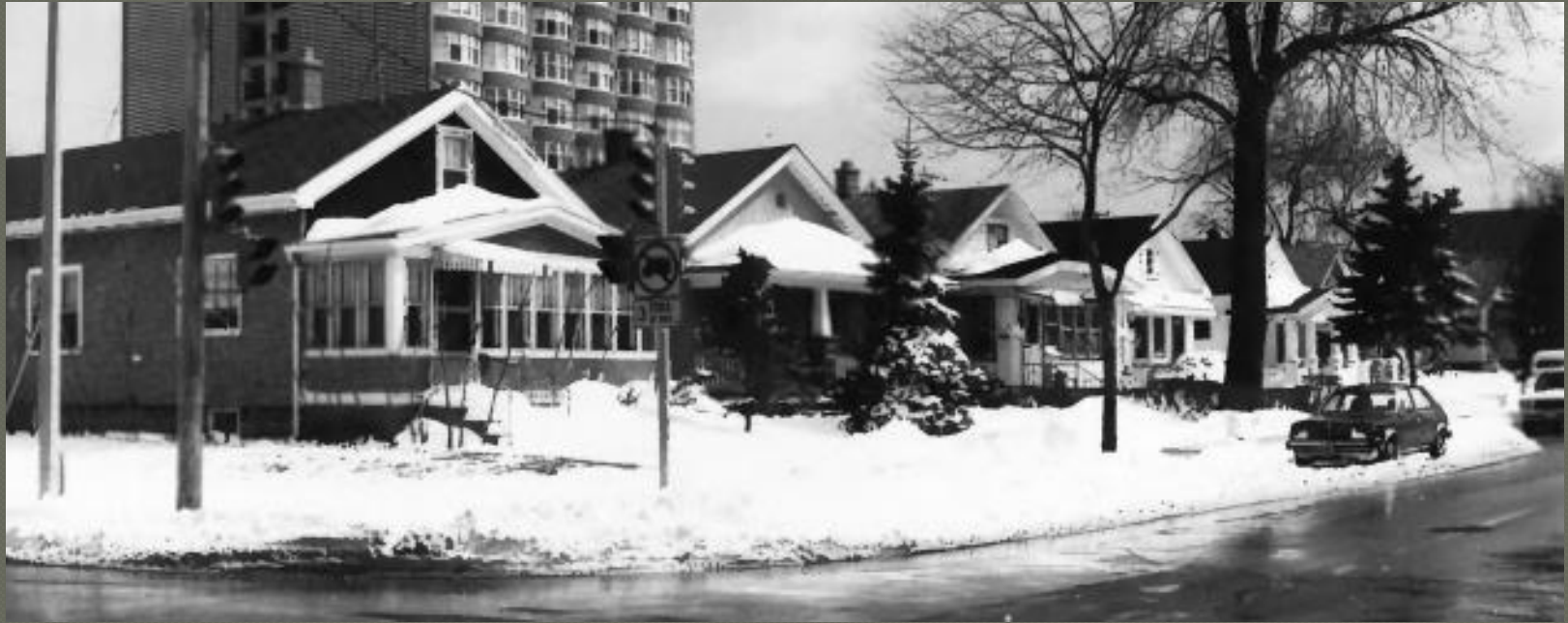
The Setting: 1982 photo of South Superior from the National Register Nomination.
