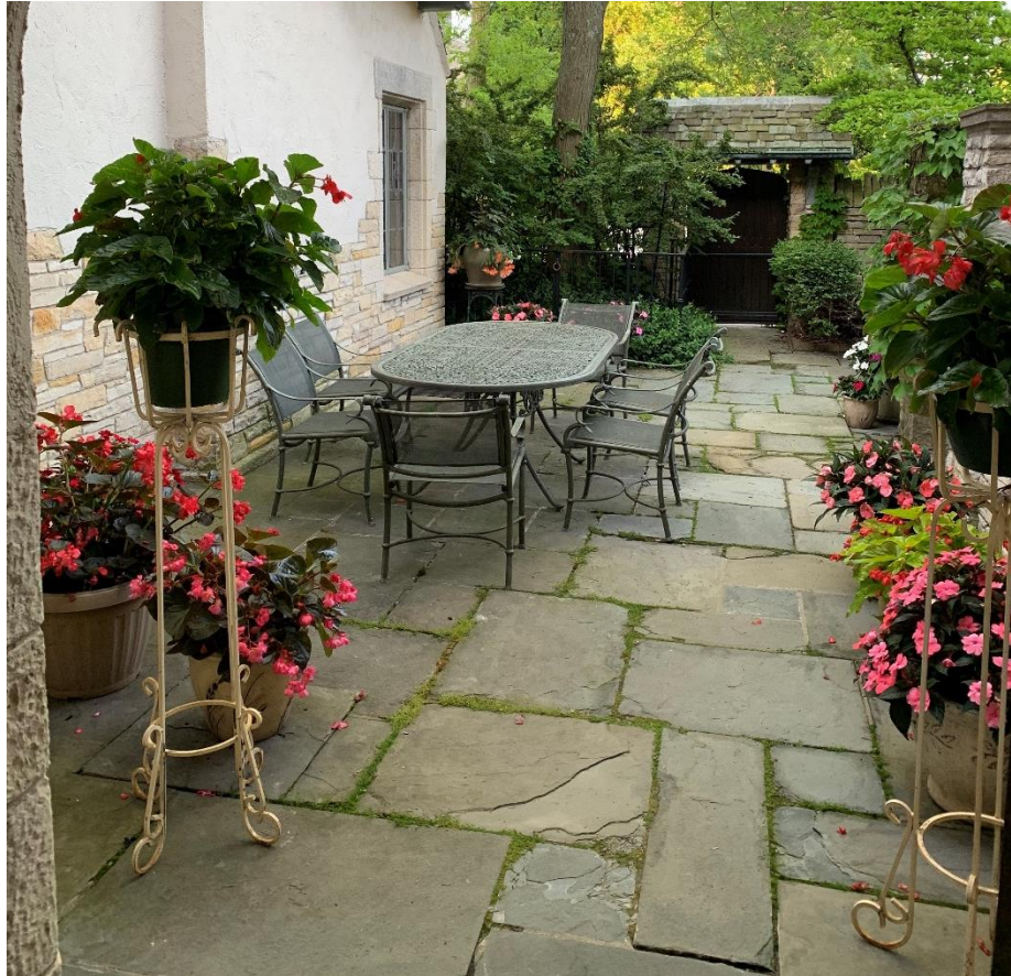
Existing patio, paver replacement in-kind
