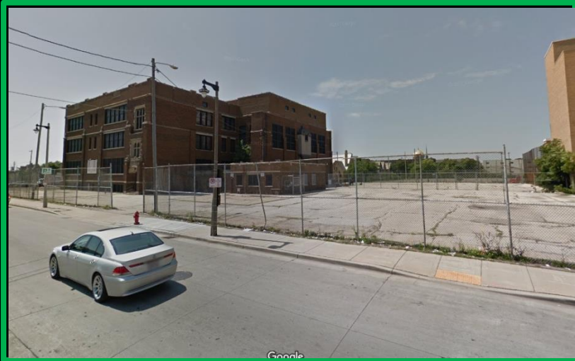
View southwest from N. 27th St. & W. Hazelton Ct.
