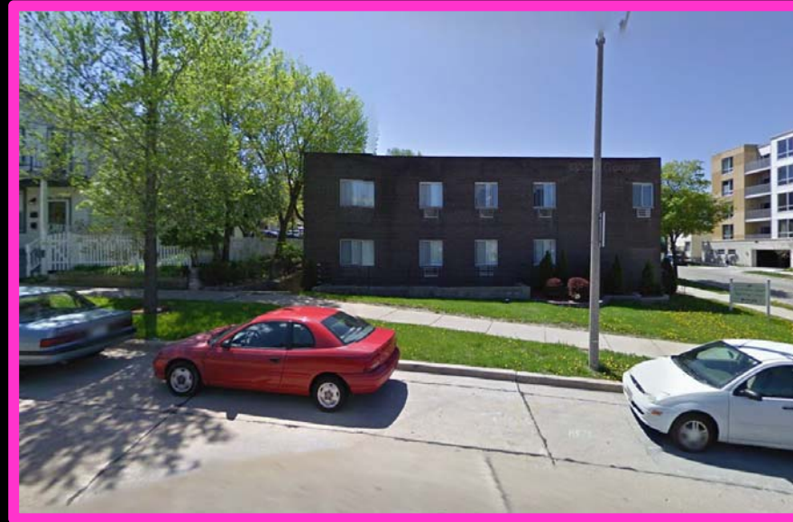
View from E. Pleasant Street looking south
