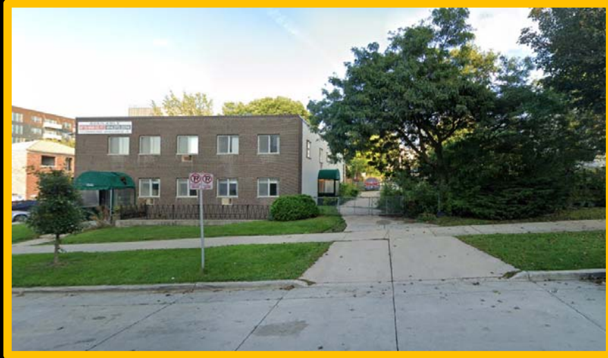
View from N. Jefferson Street looking east
