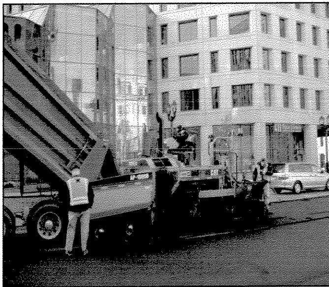
Laying the asphalt base along East Wisconsin Ave
